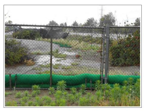
Figure 35 Filter Sox installed at San Gabriel River Nursery retains stormwater runoff from site
