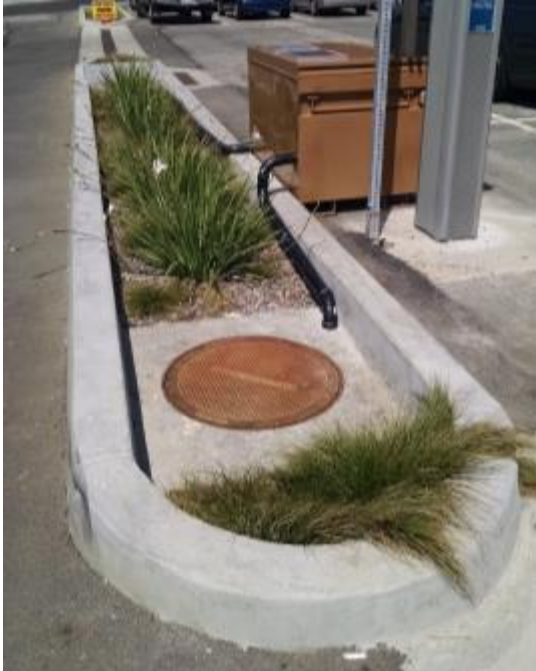
Figure 2-2 MWS No. 2 with Knack Box Equipment Housing
