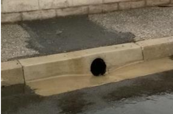
Figure 2-4 Influent Drain at Parking Lot 7
