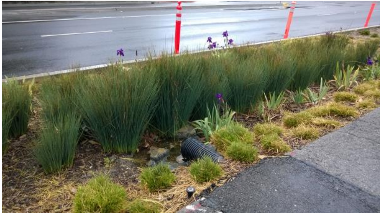
Figure 1-2 Bioretention BMP at Parking Lot 7
