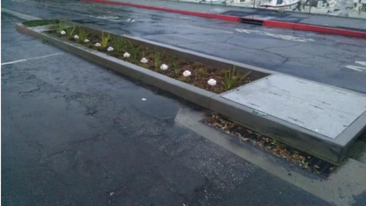
Figure 1-1 Modular Wetlands System Linear Biofiltration BMP at Parking Lot 5
