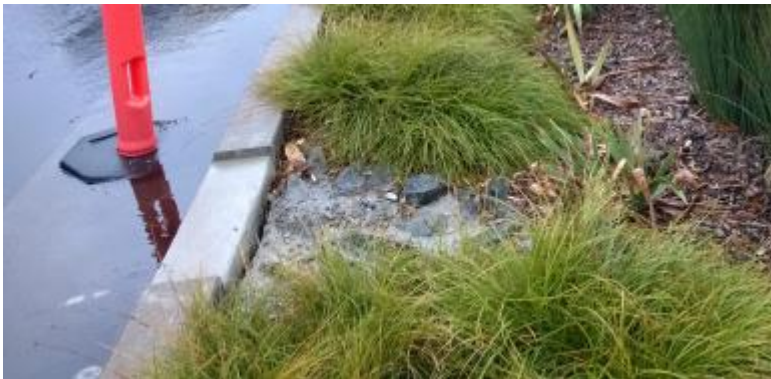
Figure 2-5 Curb Cut Out for Overflow at Parking Lot 7
