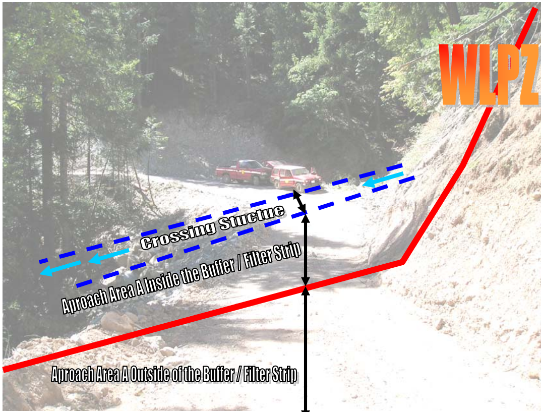
Figure 3. Approach area A inside and outside the WLPZ/ELZ. Approach area A is always on the left looking downstream.
