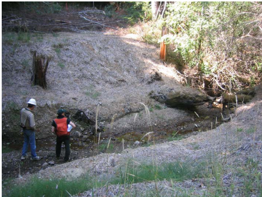
Figure 13. Pilot project Coast team members Dave Longstreth, CGS, and Richard Fitzgerald, DFG, evaluating a removed watercourse crossing in Mendocino County in August 2006.
