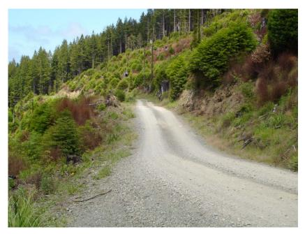
Figure 19. Example of road segment built to drain properly in wet weather. Note the two functional dips and their spacing.
