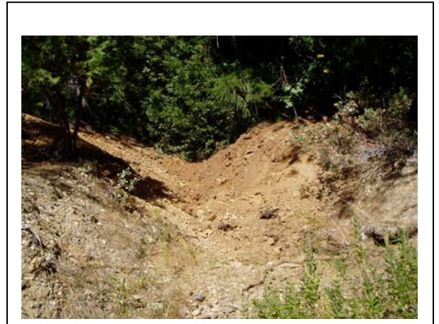
Culvert Removal "after"
