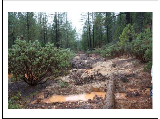
Headcut after stabilization work.
