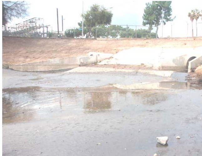
Same general area after trash capture systems installed on four outfalls
