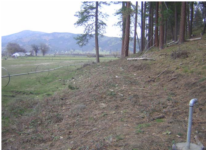
Ditch reconstruction - After
