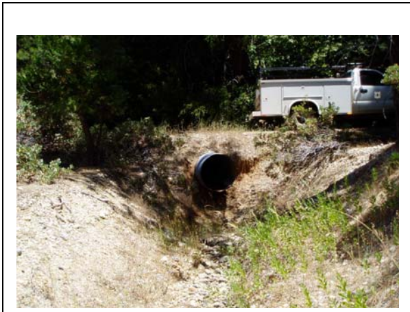
Culvert Removal "Before"
