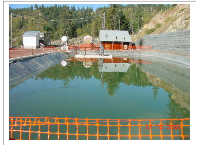
View of Klondike Settling pond before reclamation of the work pad
