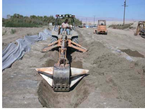
Simulated drainage ditch construction.
