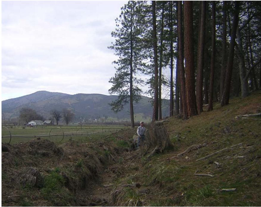
Ditch reconstruction – Before
