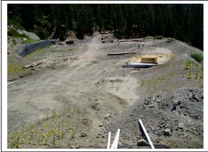
View of mine pad after demolition of the building
