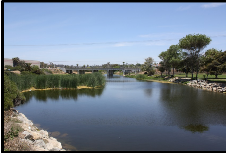
FIGURE 4 VIEW OF RIP-RAP ARMORED BANKS OF LOMA ALTA SLOUGH View to east (upstream). Photograph taken at Slough near S. Pacific Street.
