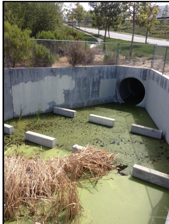
Figure 9 Loma Alta MS4 Outfall with Non-Storm Water Discharge Photograph Taken August 2013
