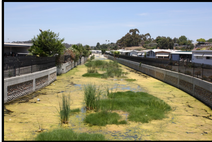
FIGURE 2 VIEW OF CONCRETE LINED SECTION OF LOMA ALTA CREEK View to east (upstream). Photograph taken at Pacific Coast Highway.
