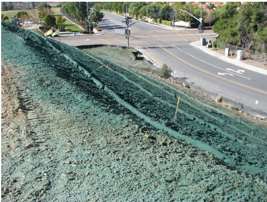
Figure 10. North slope has erosion control BMPs
