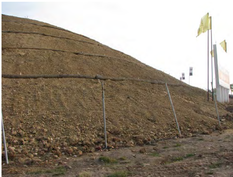
Figure 10. Slope is 2:1 Horizontal: Vertical according to SWPPP
