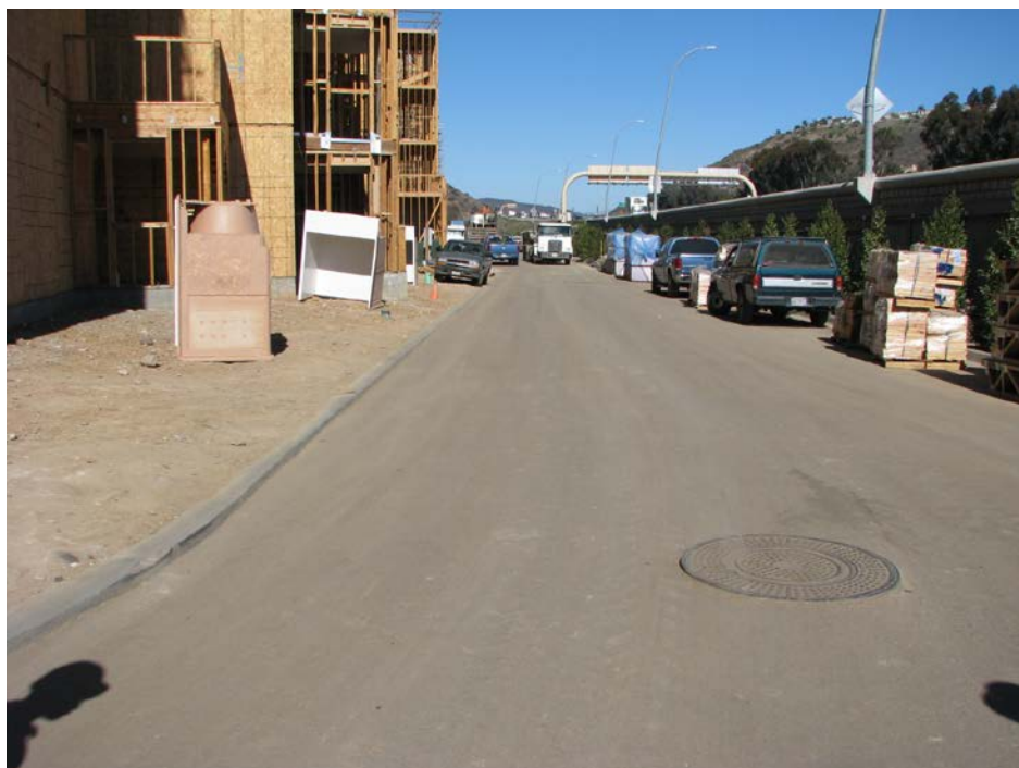
Figure 2. East side of active constructive site
