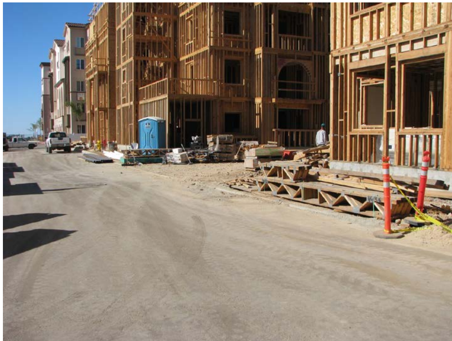
Figure 1. South side of active construction site
