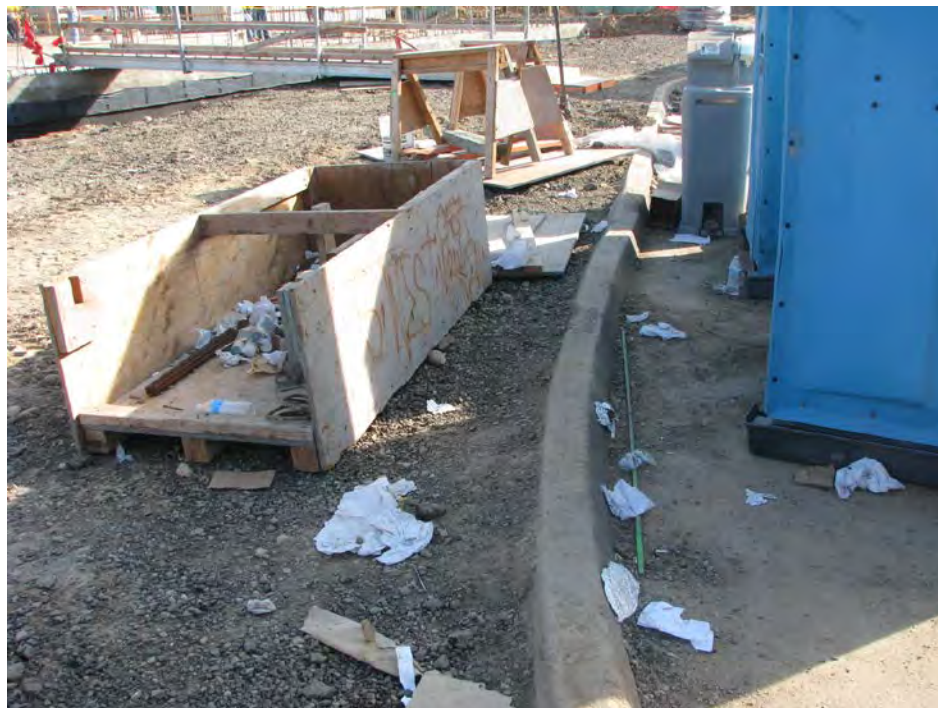
Figure 3. Site interior; trash
