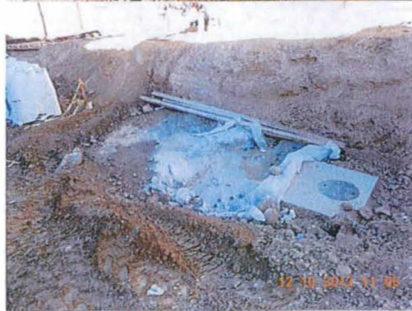
#13 Clean around Drain Inlet
