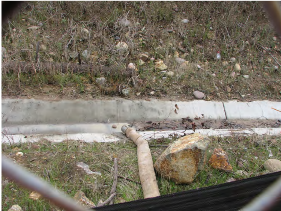
Figure 9. Outlet pipe of illegal discharge
