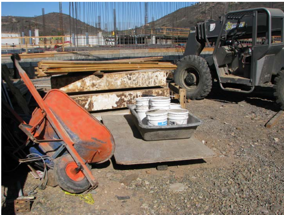
Figure 12. Chemicals with secondary containment
