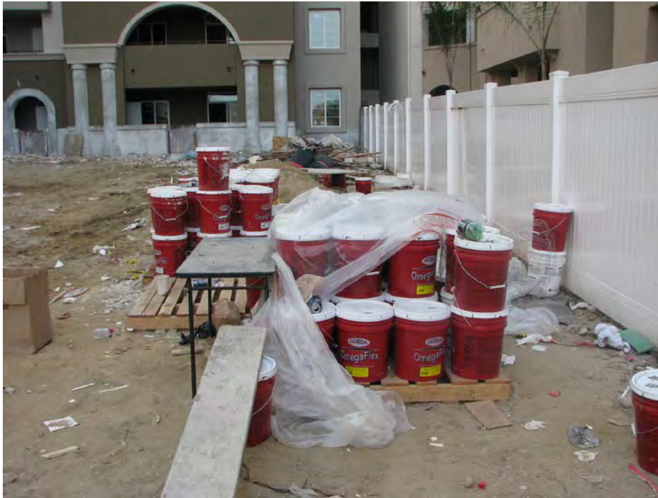
Figure 25. Improperly stored chemicals
