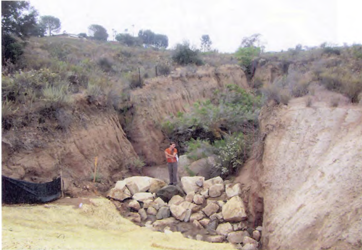
Figure 4. Ephemeral stream in highly eroded canyon, looking west from constructed off-site road knuckle. Photo by Lisa Honma, SDRWQCB, July 1, 2015.
