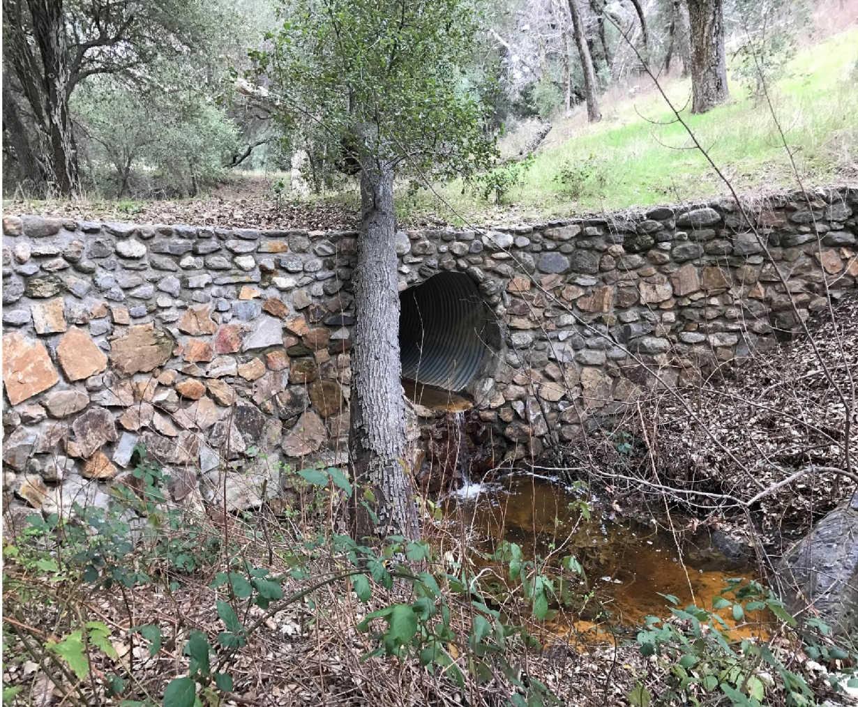
Downstream view of Stream crossing and culvert to be removed
