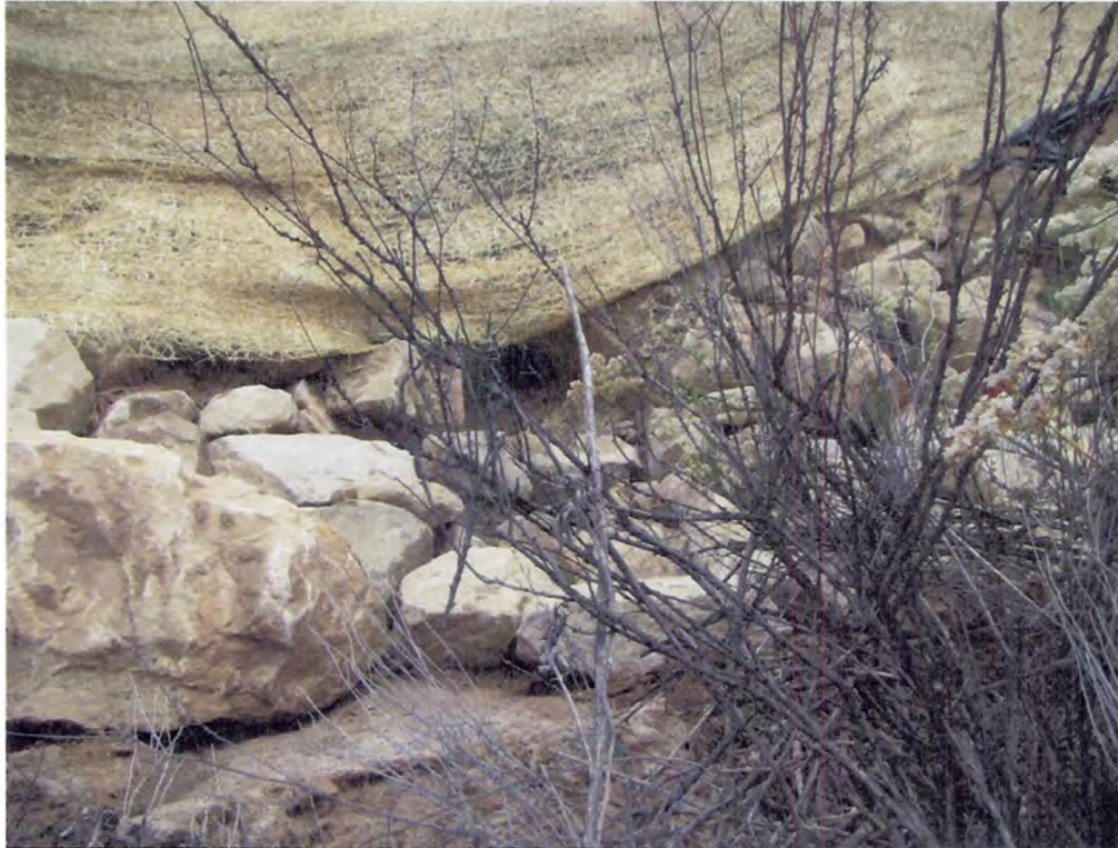
Photo 4: A second storm water inlet structure installed at the base of the fill at Drainage 2.
