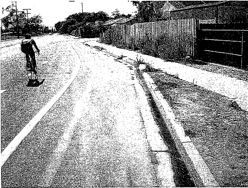
4. Dirty street before the storm drain inlet.
