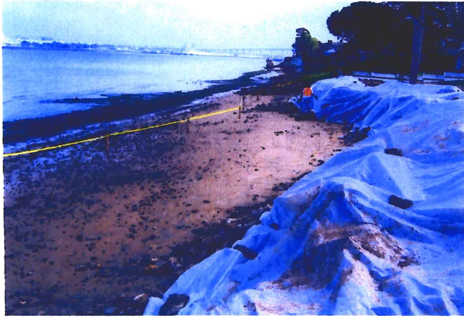
Shows end of day shore protection during rubble removal
