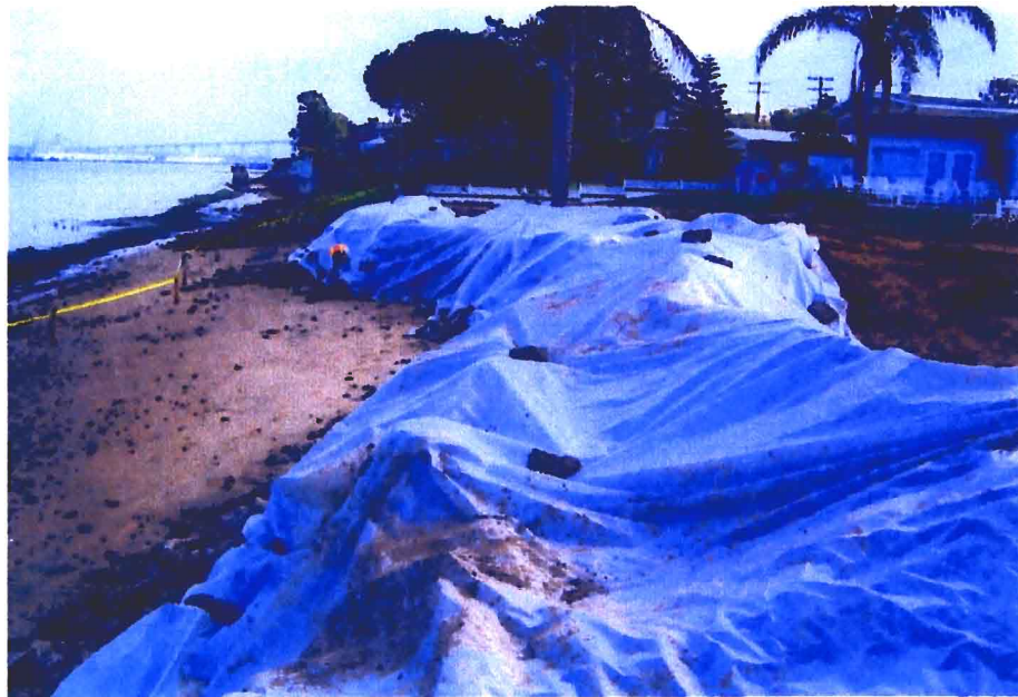
Shows end of day shore protection during rubble removal
