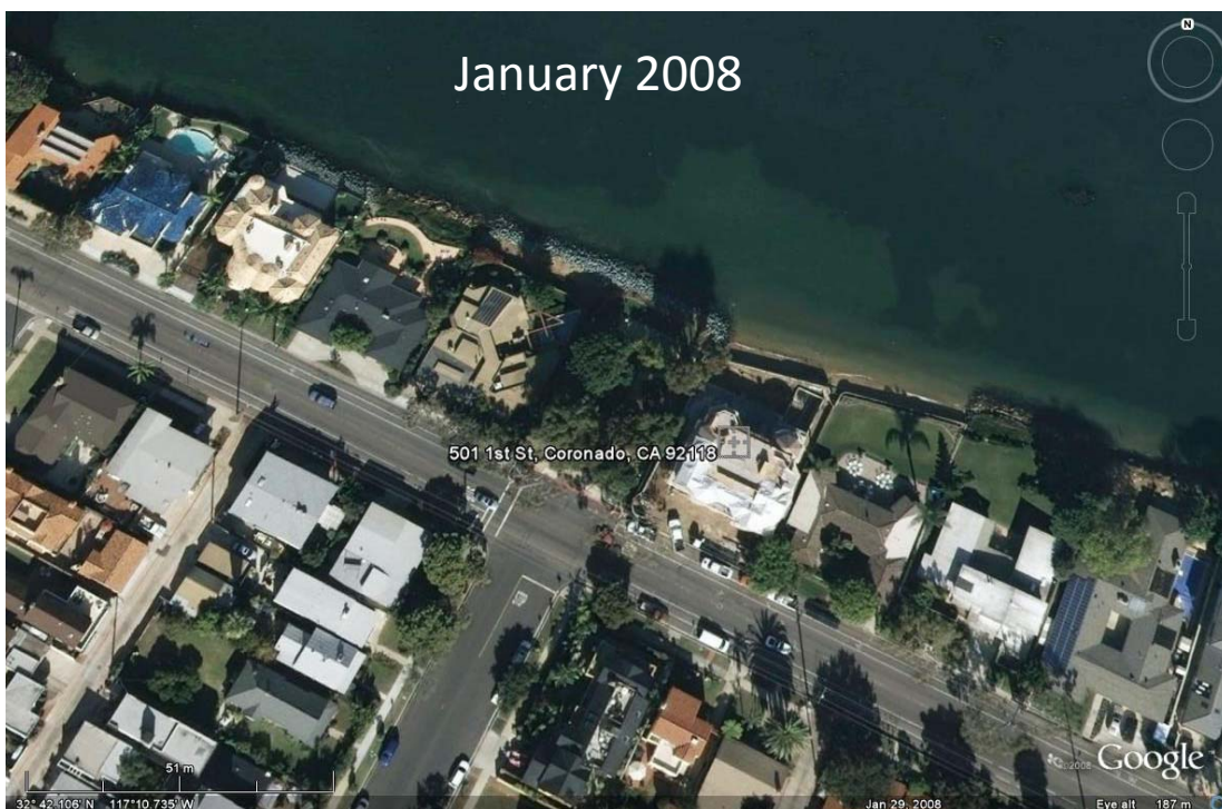
Figure 4. Photographs of 501 1 st street, Coronado, CA, taken in May 2006 (top) just after rip-rap removal and during seawall construction, and in January 2008 (bottom). Eelgrass is visible as darker areas adjacent to the shoreline.
