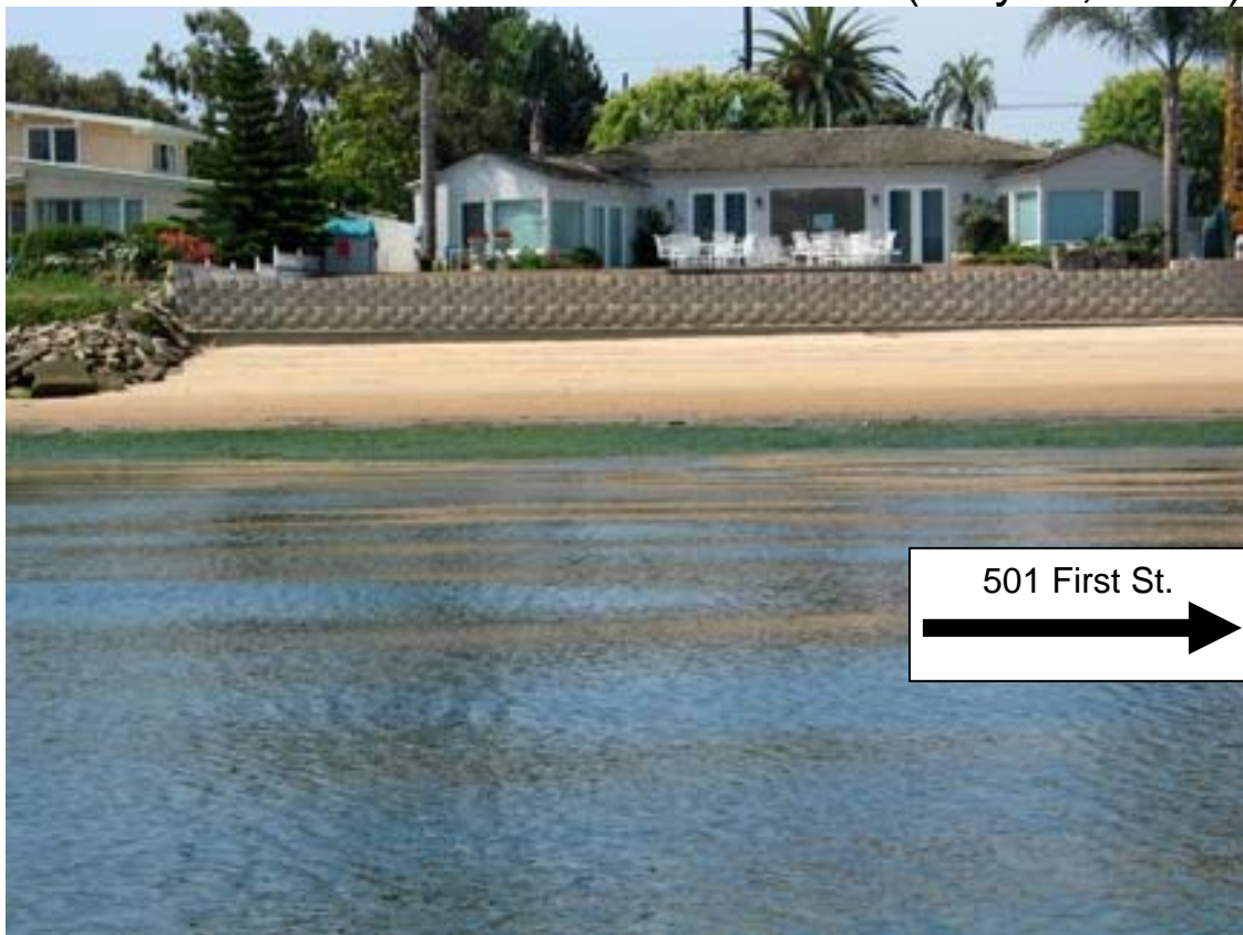
View to the southwest of 505 First St. (May19, 2006)
