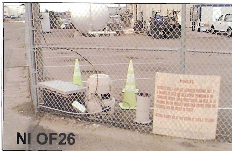
Figure 18. Naval Air Station North Island storm water monitoring location for outfall 26. The site was located along the fence surrounding a steam plant.
