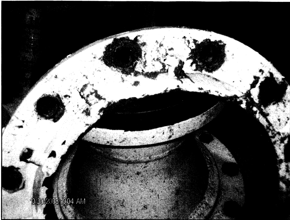
Photo #15: Pump #1 Uni-Flange Coupling (Paint on Set Screws Is Not Disturbed)
