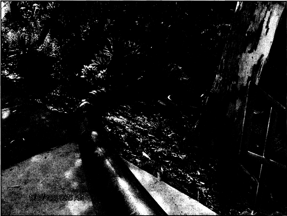
Photo #20: Bypass Pump Discharge Piping (October 30th)
