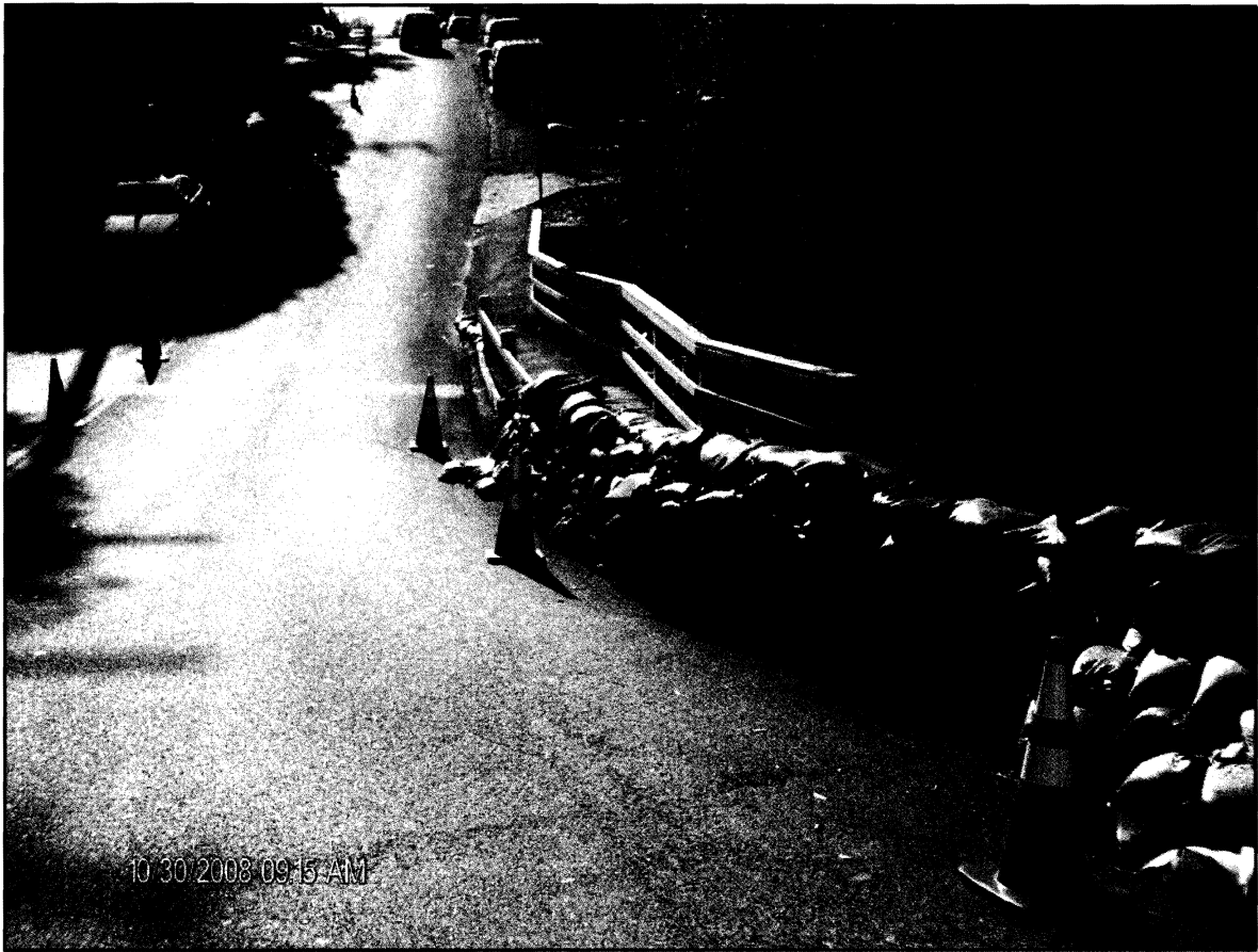
Photo #23: Traffic Control on Glenneyre Street (October 30th)
