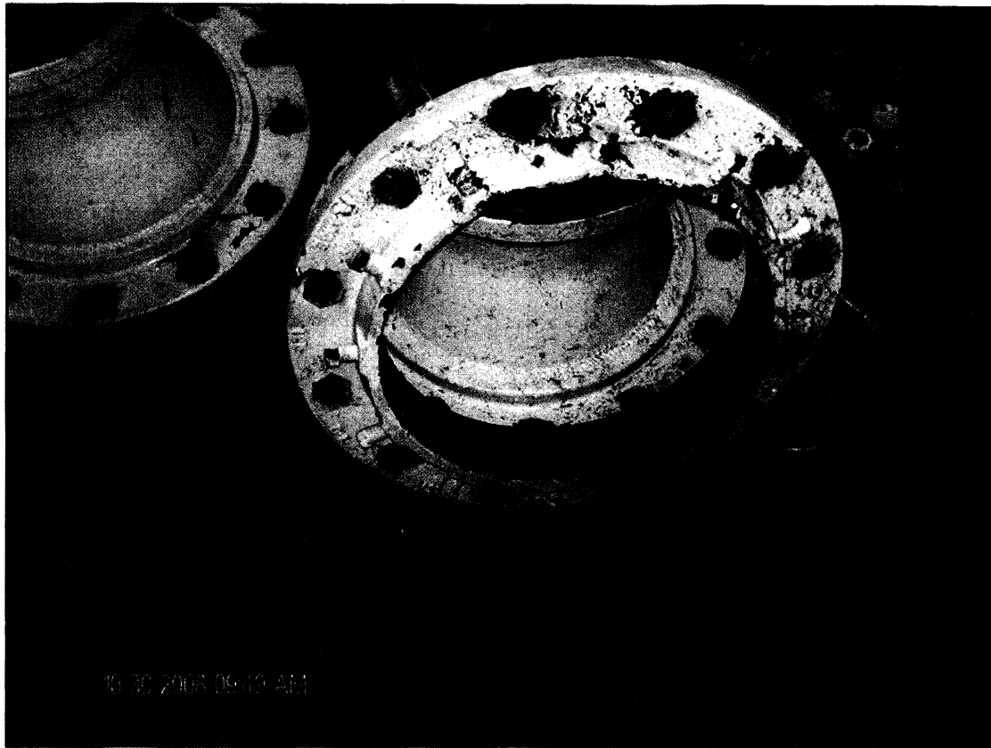
Photo #13: Pump #1 Uni-Flange Coupling
