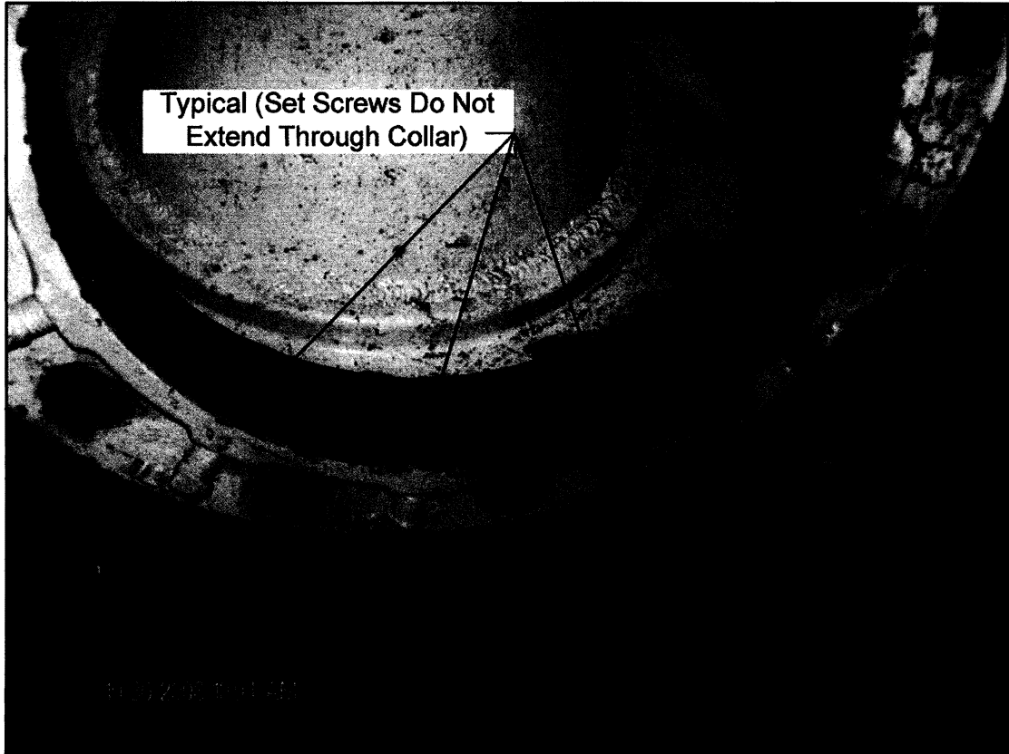
Photo #14: Pump #1 Uni-Flange Coupling (Set Screws Do Not Extend Through Collar of Coupling)
