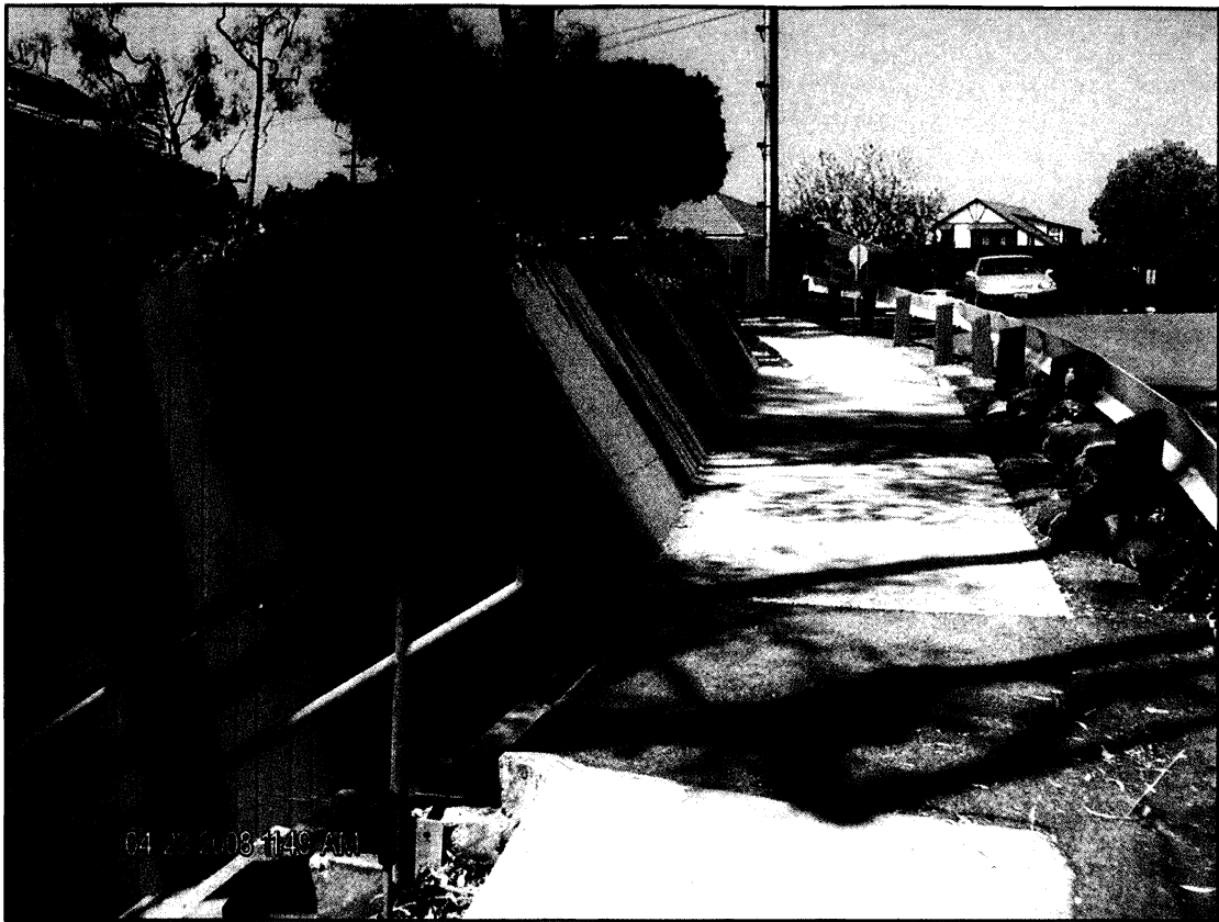
Photo #3: Pump Station Exterior (Adjacent to Glenneyre St.)
