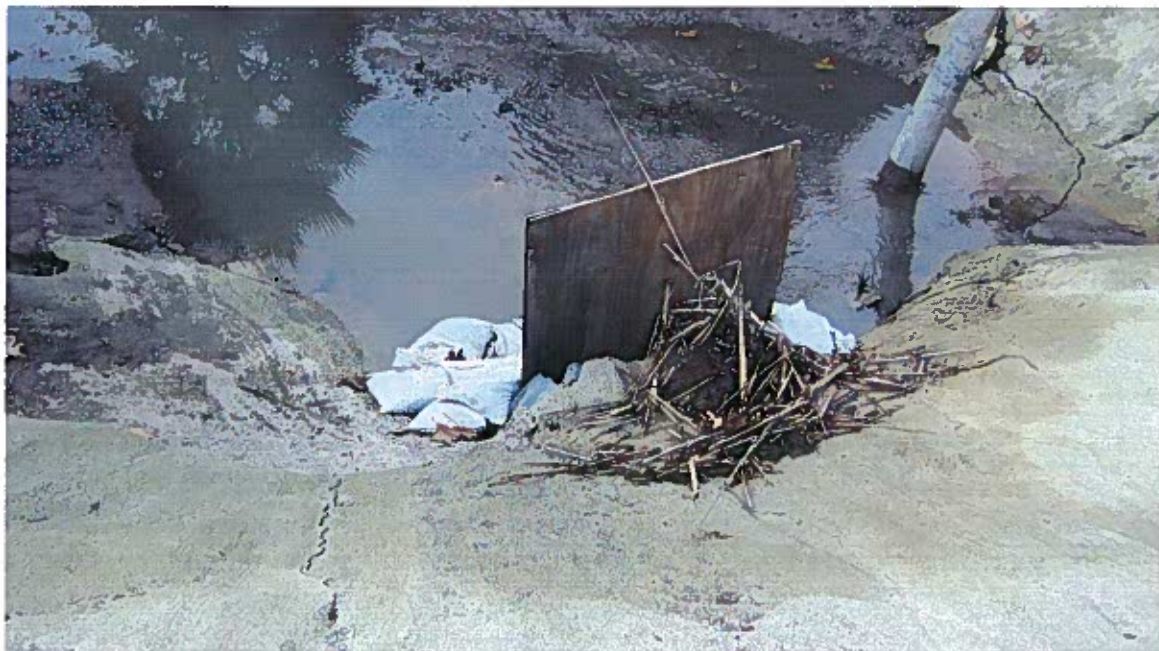
Release blocked at storm drain along Diaz Road before entering Murrieta Creek.
