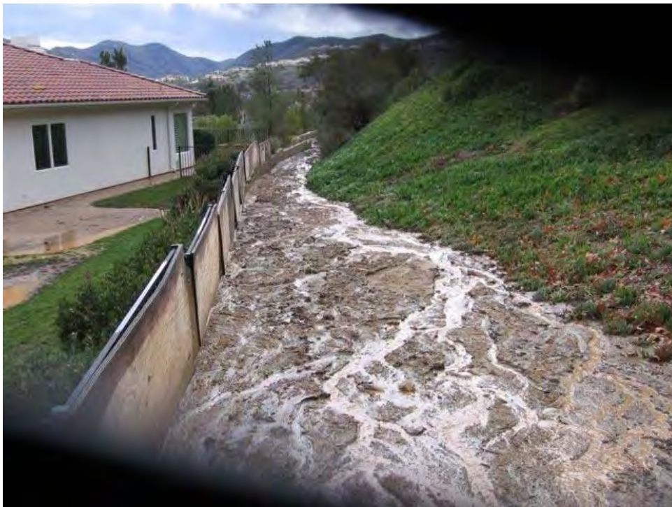
Figure 5. Photo of sediment discharge into MS4 tributary to Murrieta Creek. (IMG_005.JPG taken by County of Riverside on January 29, 2008.)
