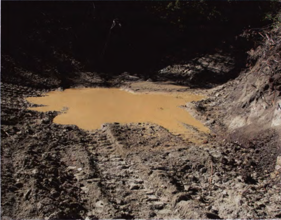
Photo 23: Natural waterway is used as a BMP. Native vegetation (Oak and some Willows) were uprooted for basin placement.
