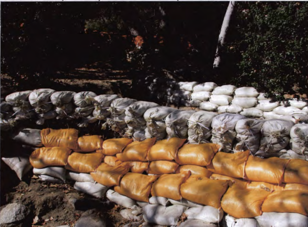
Photo 24: Fill in a natural waterway or water of the State is used as a BMP.
