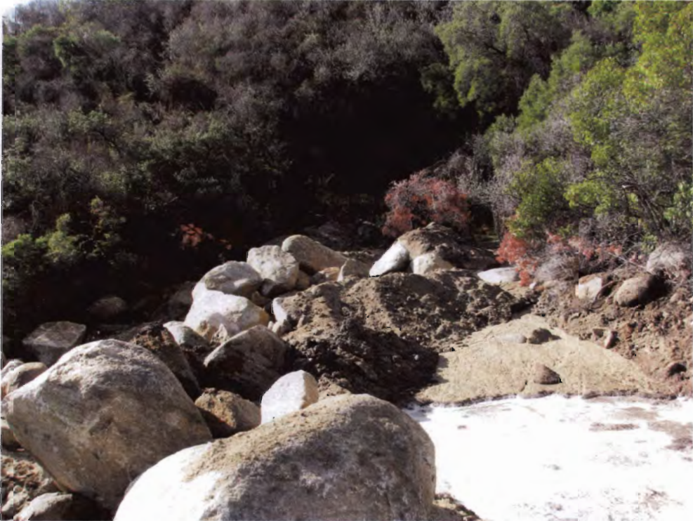
Photo 17: BMP (sediment basin) is placed within a natural waterway. Native riparian vegetation is destroyed by rocks and excavated dirt, impacting ecosystem.
