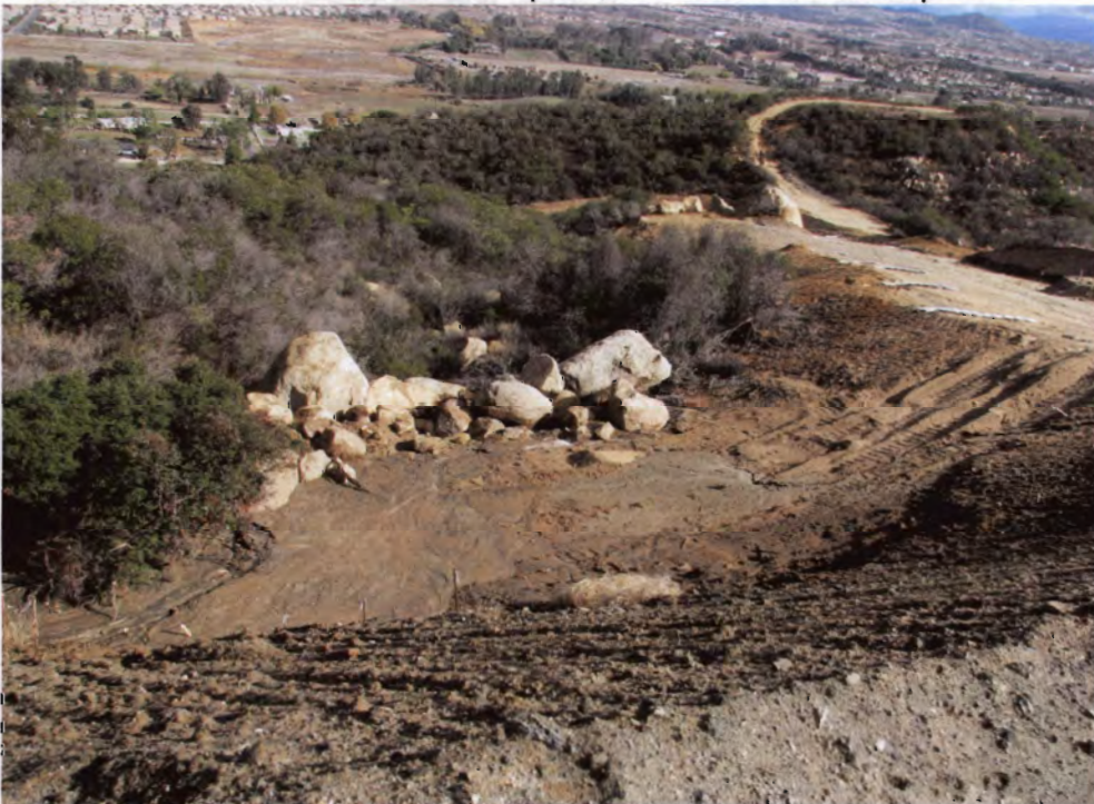
Photo 22: More fill of rocks and excavated dirt were sidescaped into natural waterway.
