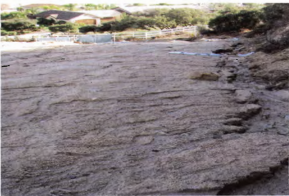
Photo 06: Erodible slopes and sediment buildup on fire-road from recent rains
