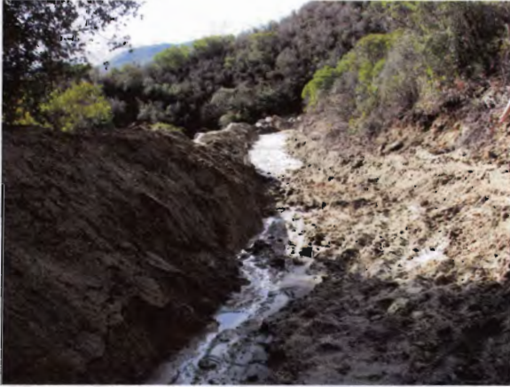
Photo 16: Shows erodible slopes leading to sediment basin
