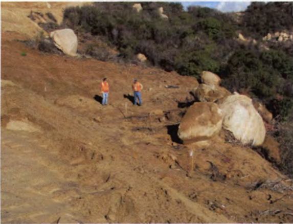
Photo 11: Construction fill (sediment, silt, rocks, and boulders) dumped in waterway (two inspectors are standing waterway)
