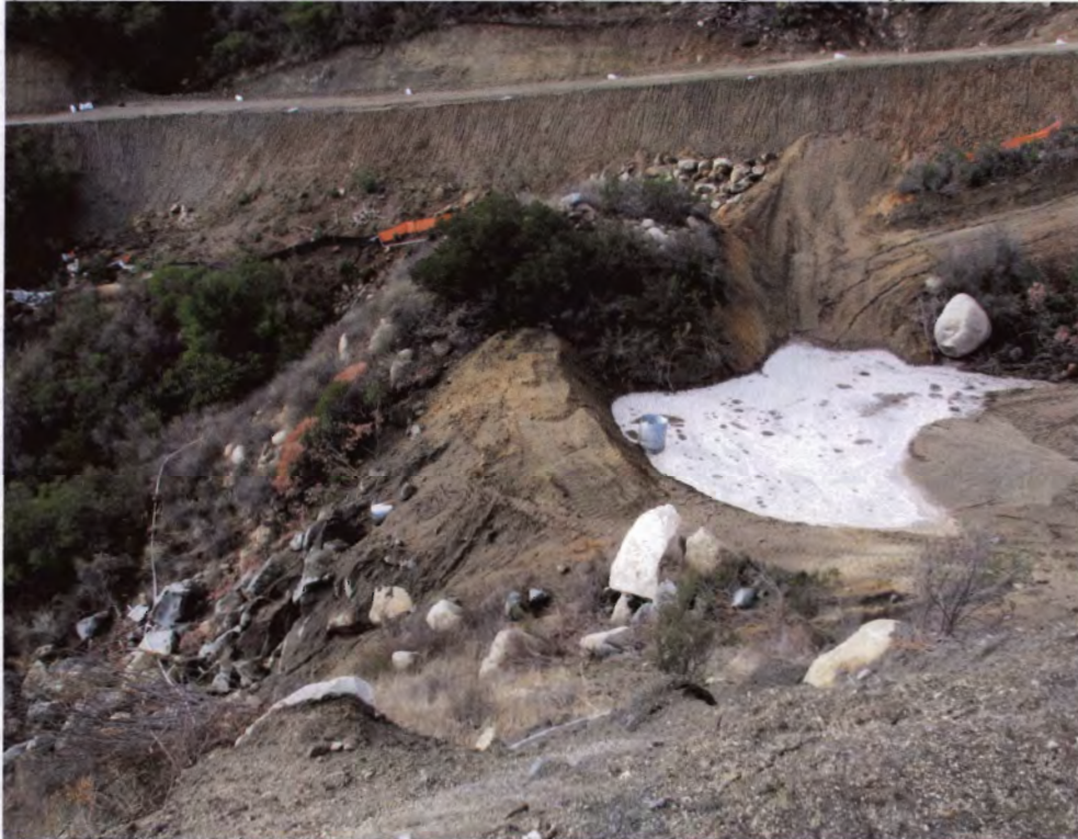
Photo 21: Third basin is built in a natural waterway or water of the State. Flow from this basin connects with the previous basin shown in photo 17.
