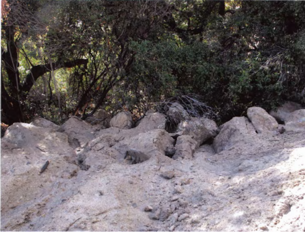
Photo 15: Rocks and dirt are sidescaped into a natural waterway (Water of the State). Discharge is to the hardened channel flowing to Bear Creek.
