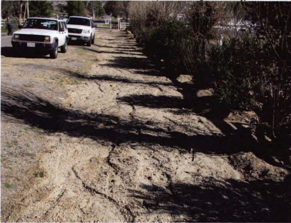
Photo 03: Looking east-shows the extent of offsite sediment discharge reaches along Claremont Street.
