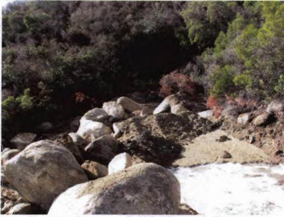
Photo 19: Close-up of fill in waterway
