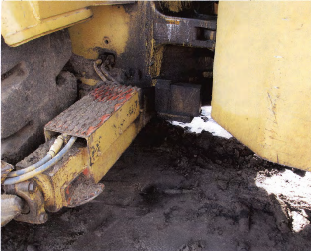
Photo 29: More spills or leaks from construction vehicle.
