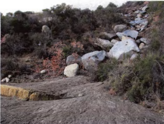
Photo 23: Rocks, sediment and silt deposited in natural drainage
