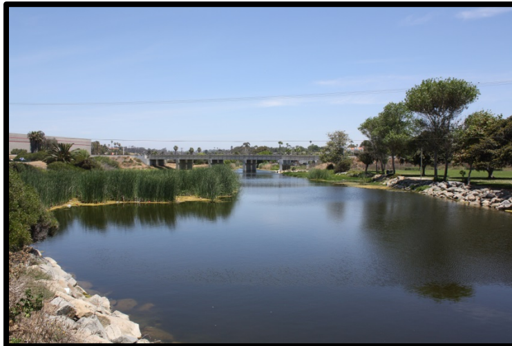
FIGURE 4 VIEW OF RIP-RAP ARMORED BANKS OF LOMA ALTA SLOUGH View to east (upstream). Photograph taken at Slough near S. Pacific Street.
