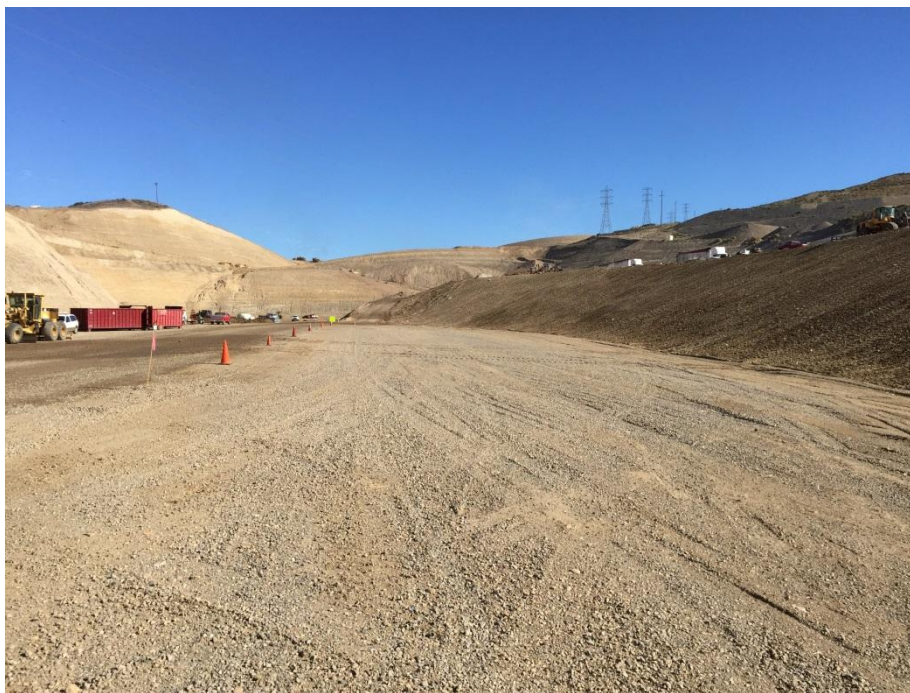
Figure 1: The new Stage III-D2 unit at Sycamore Landfill
