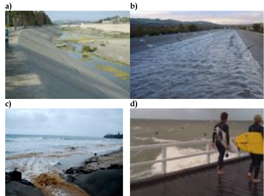
Figure 2.3.10: Photographs showing examples of the changes in flows during dry and wet weather and the subsequent changes in ocean water quality. a) Dry weather flows are much smaller than b) wet weather flows; c) wet weather flows from stormdrains and channels typically reach the ocean in wet weather, in contrast to dry weather flows which rarely reach the ocean; d) surfers often take advantage of the large waves caused by winter storms, despite the increased exposure to contamination this may involve.
