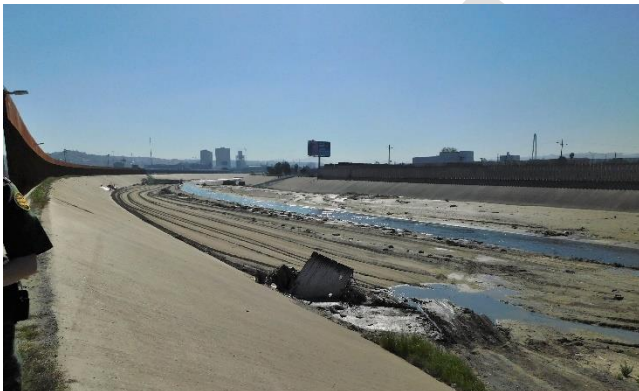
Lined portion of Tijuana River Flood Control Channel (facing upstream)
