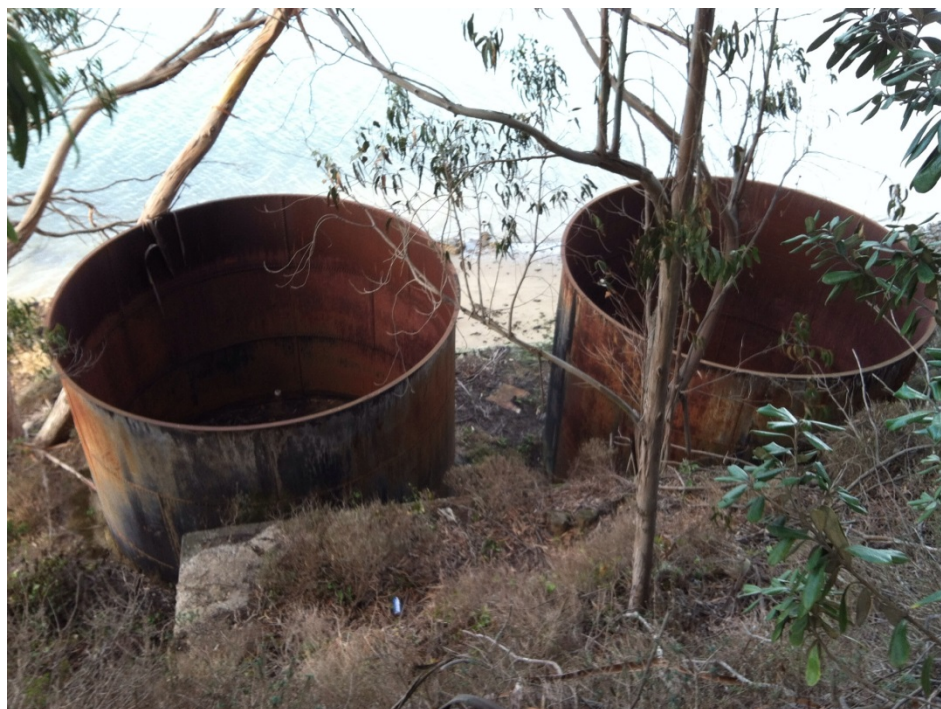
Figure 1b. Former fuel storage tanks for steam plant operation.
