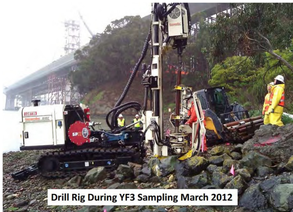
Figure 1c. View of drill rig used during March 2012 sampling event.
