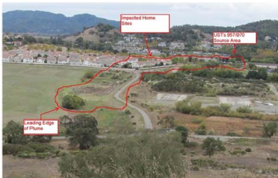
Photo 3. Petroleum release source area, extent of MTBE plume, and residential development location.
