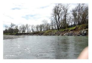
**Figure 3:** This photo is of the same stretch of project following the first high velocity flow event that the project experienced. It is clearly seen here that all the vegetation was removed during that high velocity event and the bank was further degraded.
