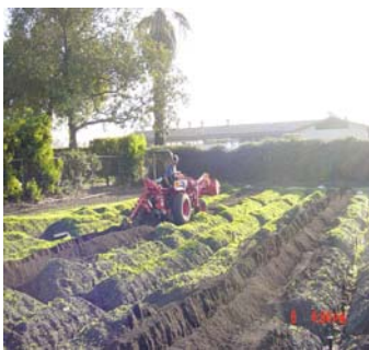
Photo1. Irrigation trenches being dug
