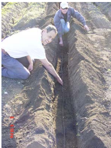
Photo 3. Aquaflex ® sensors being installed in each plot
