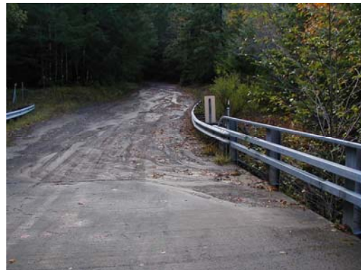
Figure 2 Road sediment draining to stream
