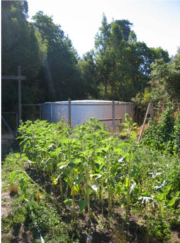
Figure 1: Completed 30,000 gallon cistern that will serve to irrigate the Organic Garden Project using water captured from the lunch shelter roof.
