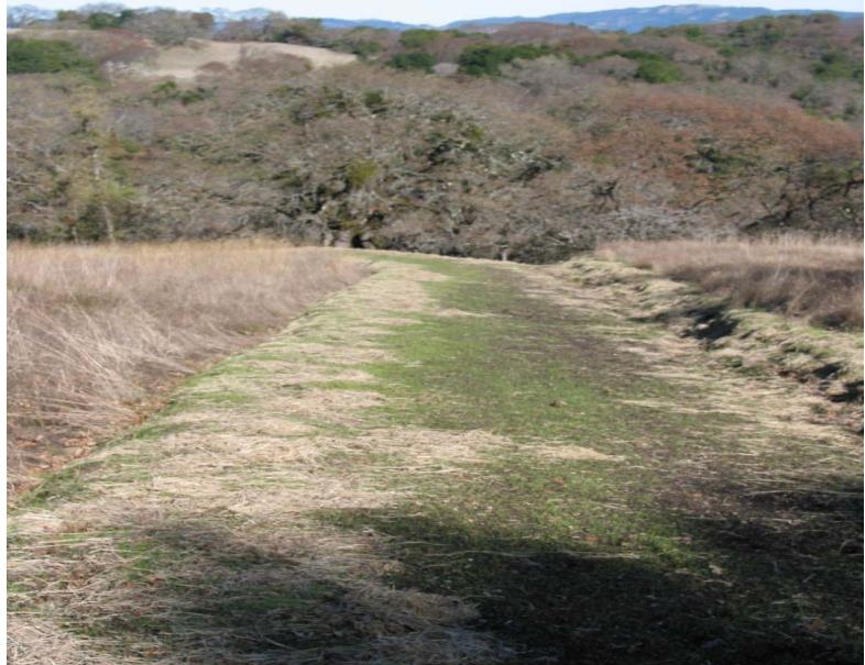
Figure 3. Re-contoured Roadbed. Erosion Control Materials Placed and Grass Cover Growing.
