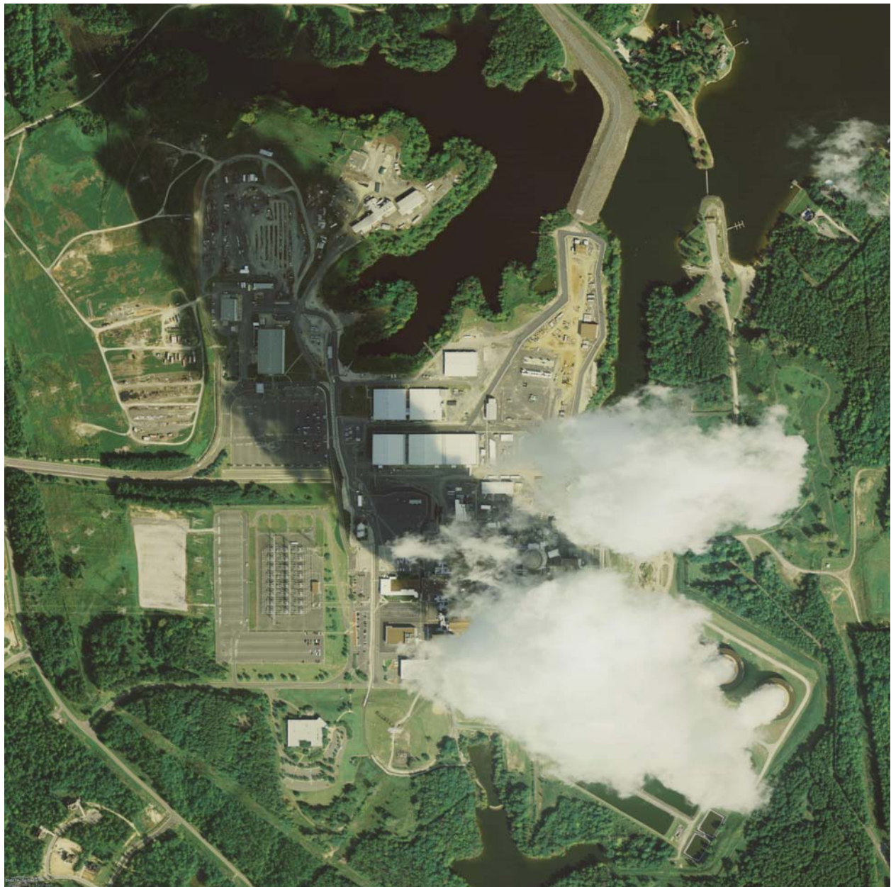
Figure 5-6 Plume Emitted from Catawba Nuclear Station (Dry-Bulb: 65°F, Relative Humidity: 90%)
