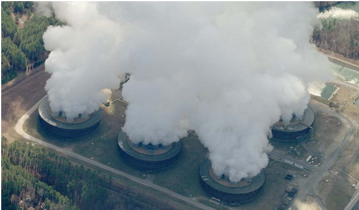
Figure 5-9 Bird's Eye View of Catawba's Non-Plume-Abated Mechanical Draft Cooling Towers (3 of 3)
