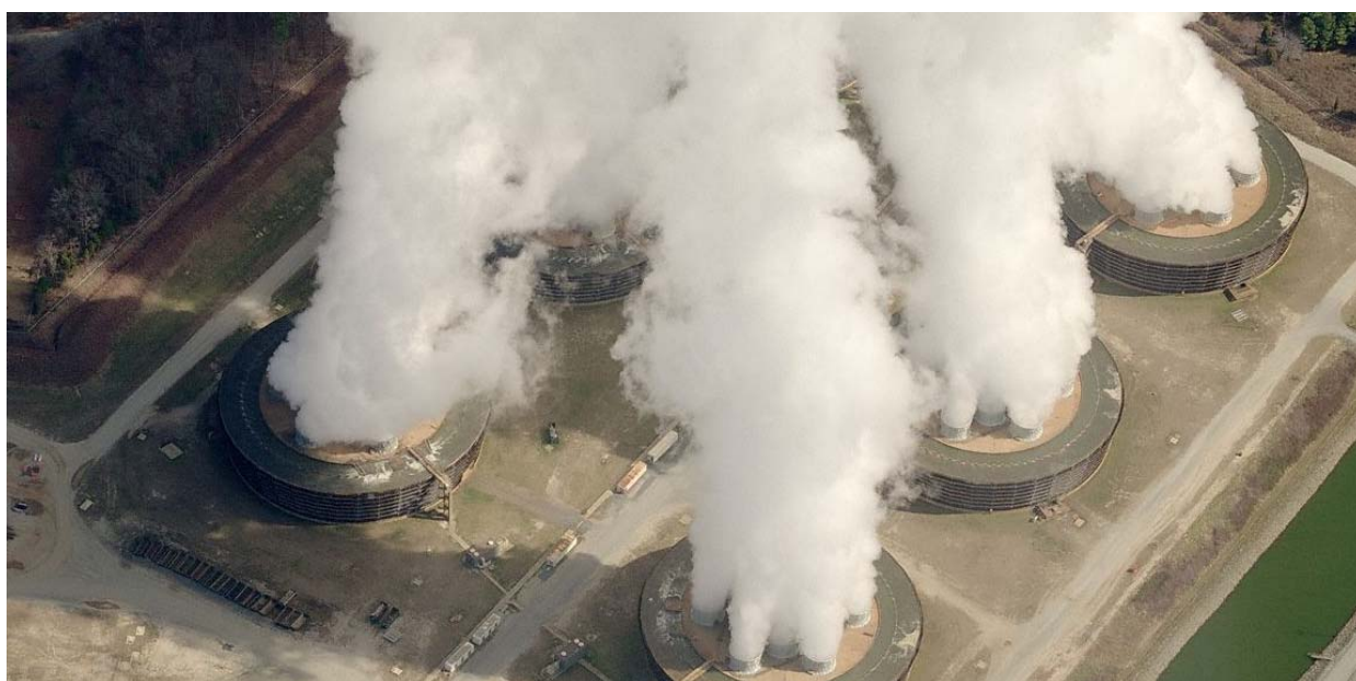
Figure 5-8 Bird's Eye View of Catawba's Non-Plume-Abated Mechanical Draft Cooling Towers (2 of 3)
