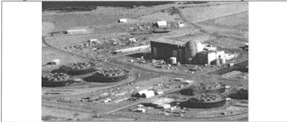
Figure 9. Palo Verde Nuclear Plant with Round Mechanical Draft Cooling Towers 55
