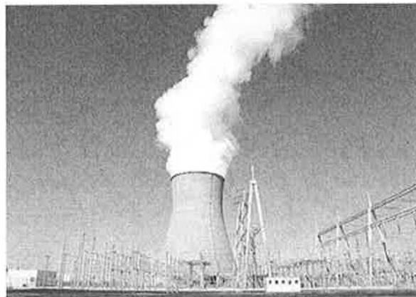
Figure 10. Hope Creek Cooling Tower 56
