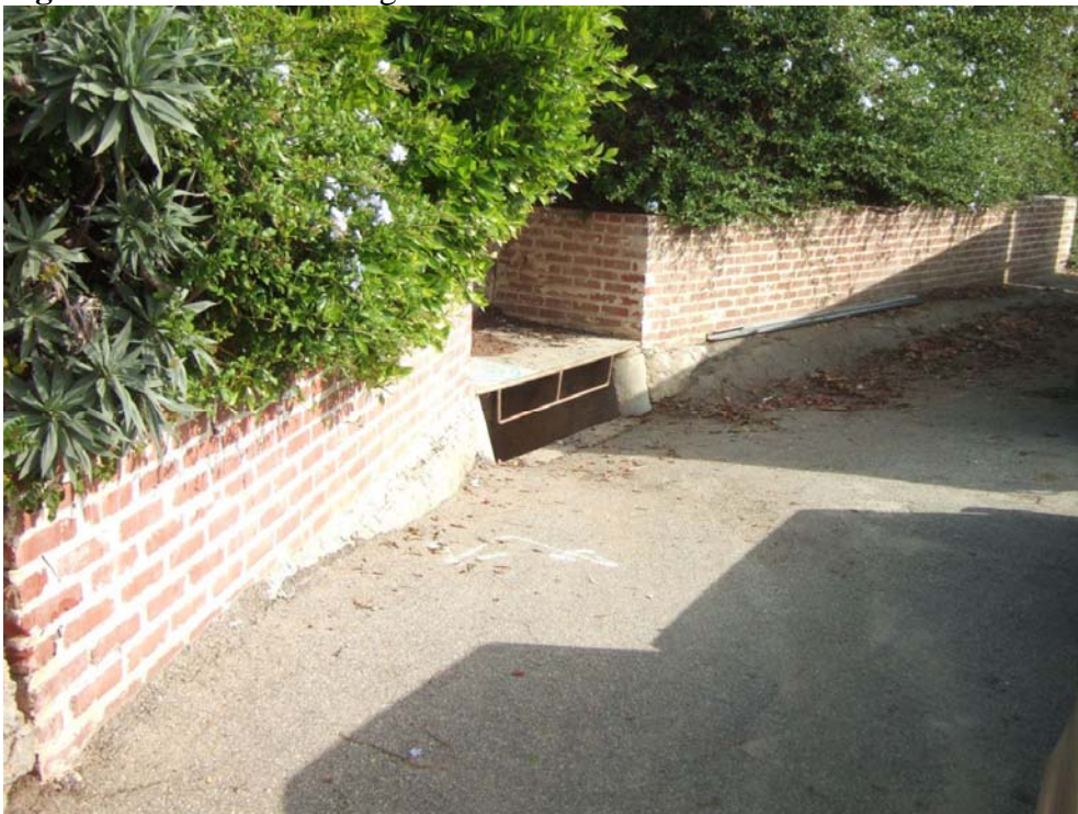
Figure 2-8. Brick retaining wall
