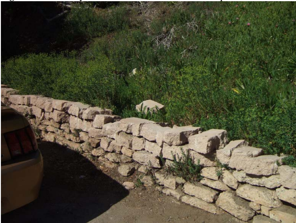
Figure 2-7. Privately constructed waste concrete hardscape
