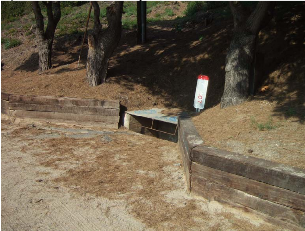
Figure 2-9. Treated wood retaining wall
