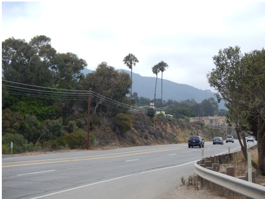
Figure 7-8. Directly Above Broad Beach Area
