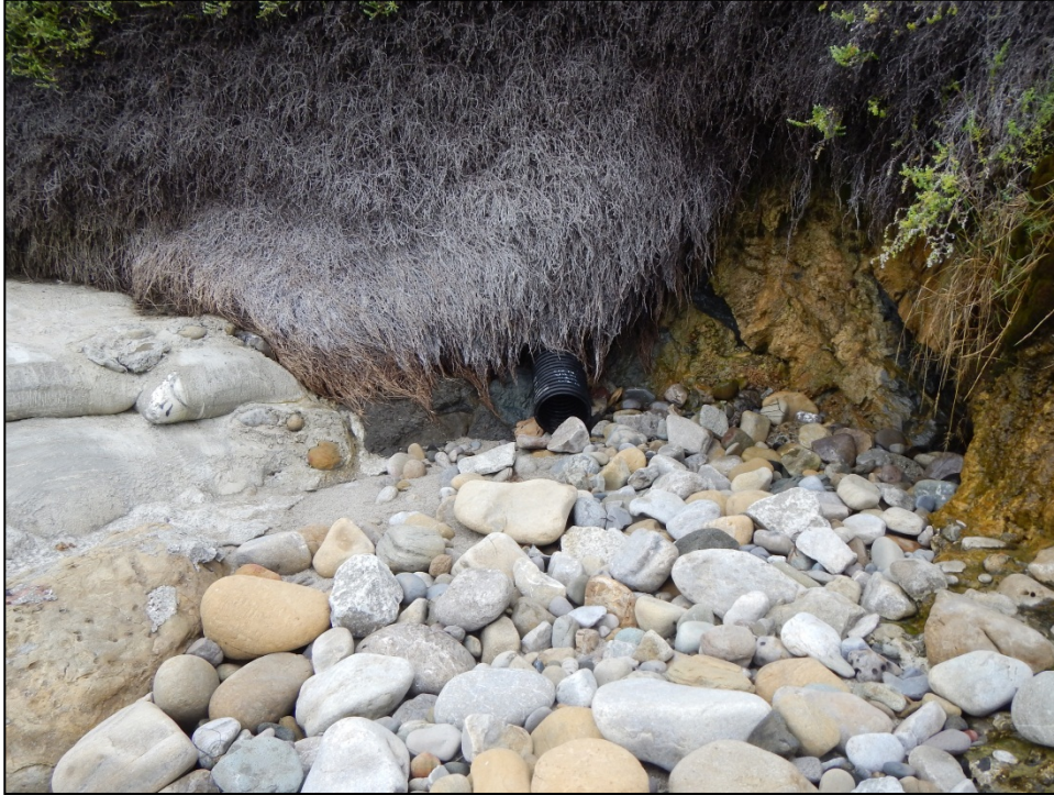
Figure 2-11. Typical Residential Small Drain Near La Piedra State Beach (ID #MUG151, 6-Inch Diameter)
