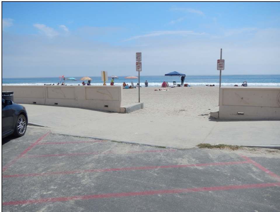
Figure 2-9. Typical Parking Lot Low Point/Sheet Flow Conveyance at Zuma County Beach (ID #MUG237)
