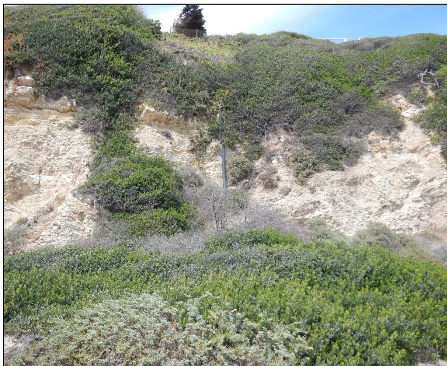
Figure 2-16. Typical Residential Small Drain Near Westward County Beach (ID #MUG393, 4-Inch Diameter)
