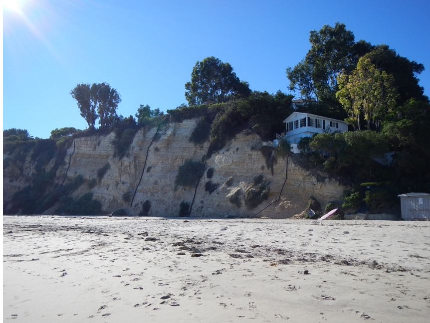
Figure 7-18. Private Drain in Little Dume Area (Typical)
