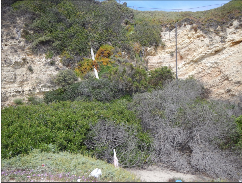
Figure 2-15. Typical Residential Small Drain Near Westward County Beach (ID #MUG437 & 438, 4-Inch Diameters)
