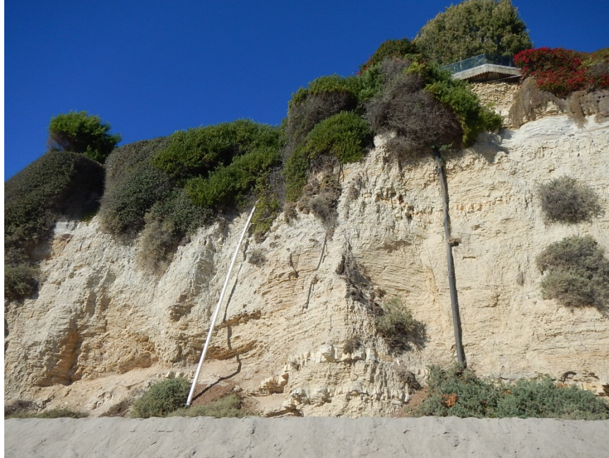
Figure 7-16. Private Drains Located in Point Dume (Typical)
