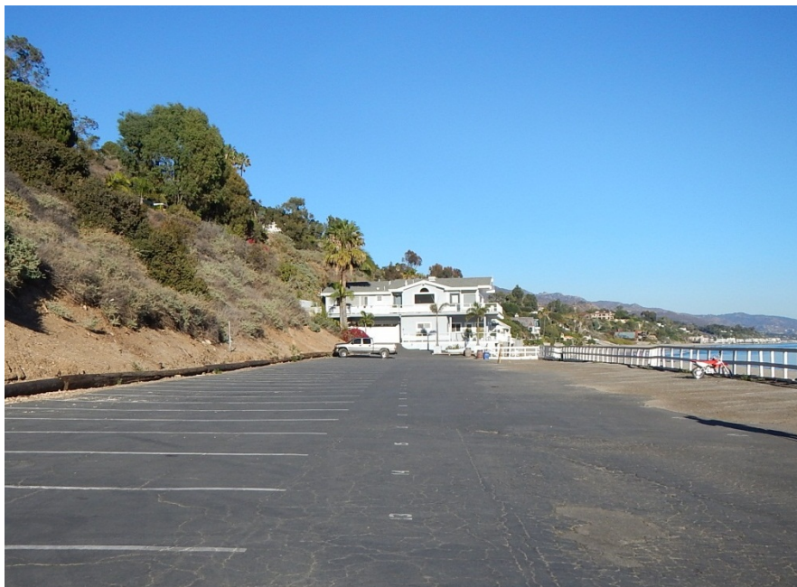
Figure 7-19. Parking Lot and Sloped Area at Paradise Cove
