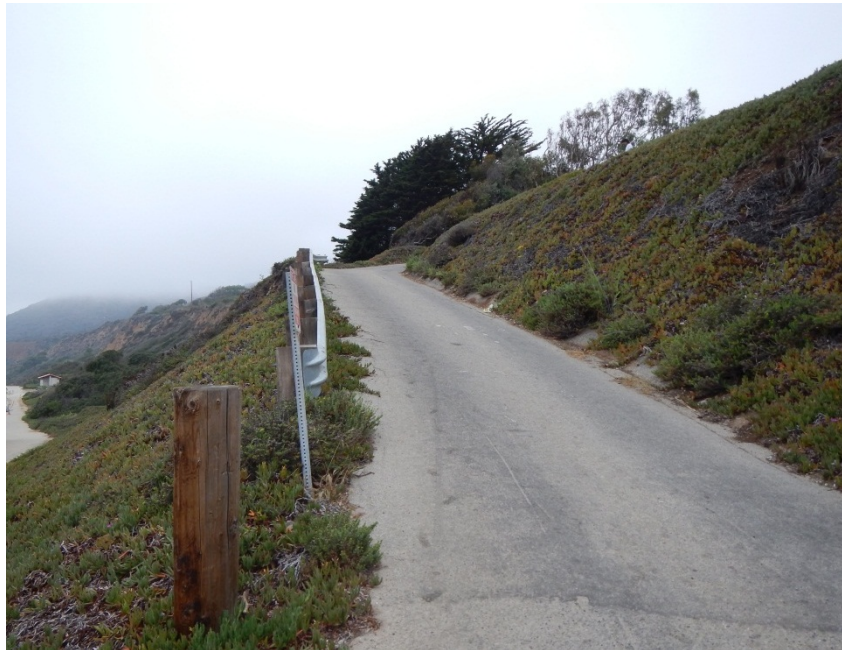
Figure 7-6. Nicholas Canyon County Beach Access Road and Slopes
