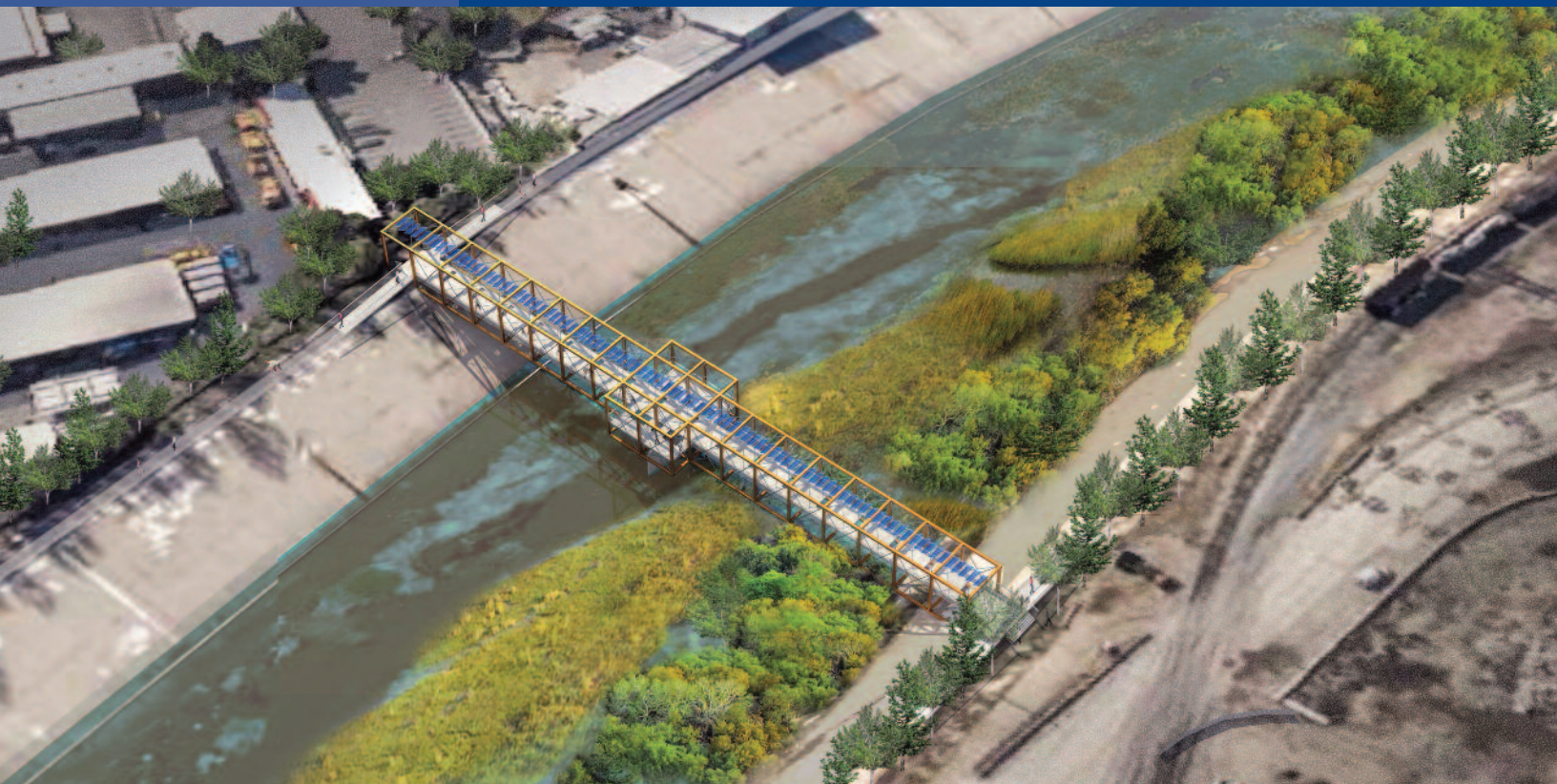
The Taylor Yards Crossing Community Bridge, proposed by Studio Pali Fekete architects [SPF:a]
