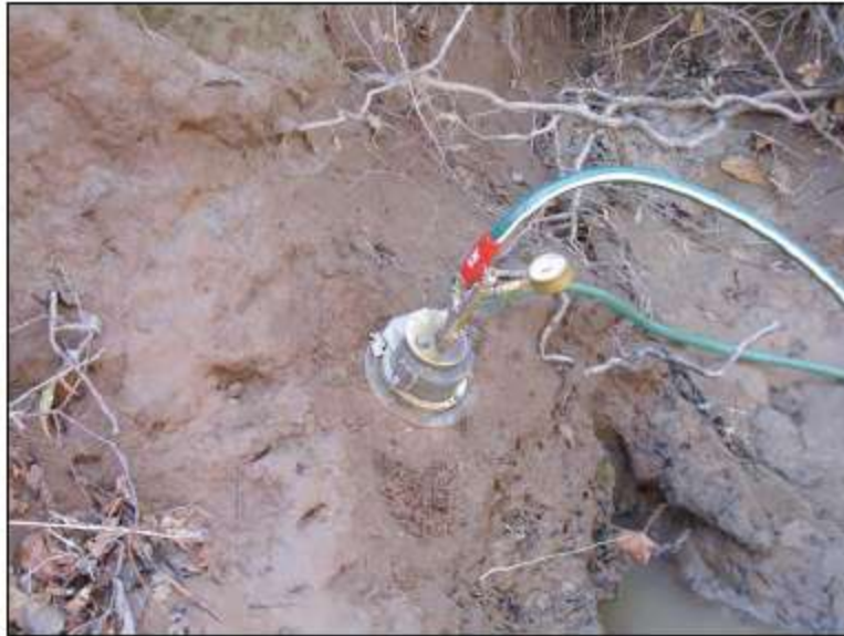
Typical installation of jet testing equipment in stream bank
