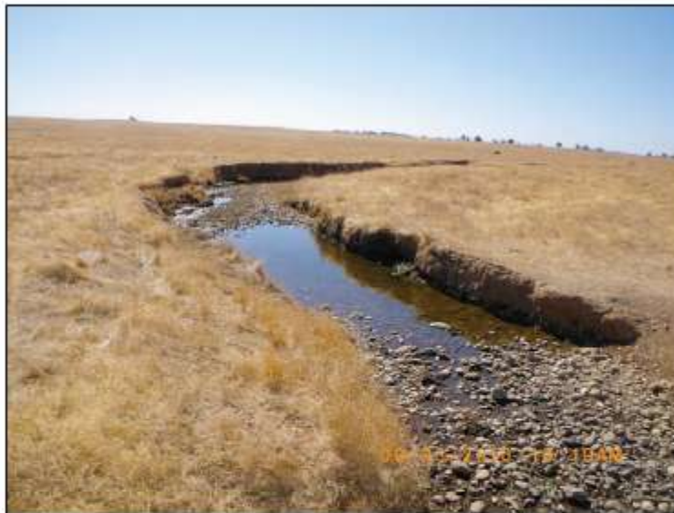
Typical stream erosion in a northern California stream (generally cohesive silty clays) (Photo cbec, inc.)
