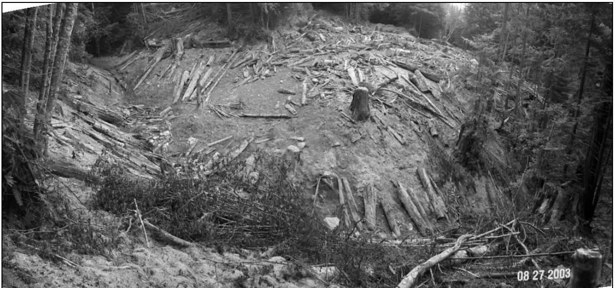
Figure X-D-19. Site # 3, 1311 Road, after excavation. This is a 2 shot panoramic compilation photo taken from near the same location as the previous picture. The site has been completely excavated, large woody debris removed from the fill during the excavation has been redistributed along the stream crossing slopes and seed & mulch has been applied to the bare slope areas.
