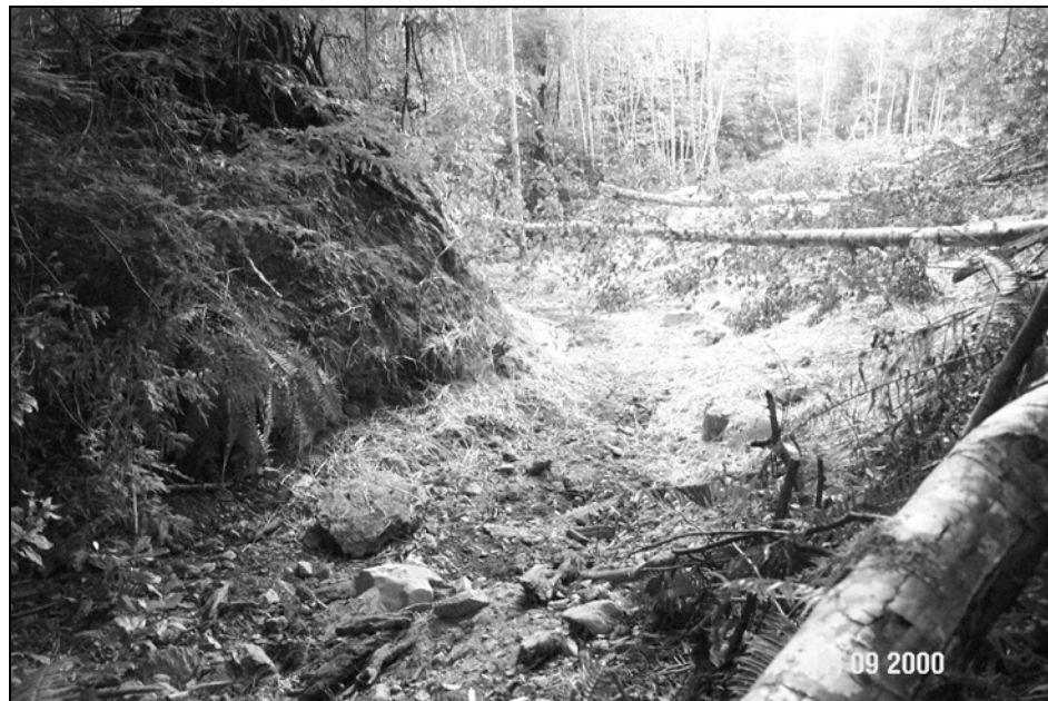
Figure X-D-5. Site #8, 1300 Road, after excavation. This picture was taken from the same viewpoint as above. The stream crossing has been excavated, mulched and seeded. See same view below after heavy rainfall (Figure X-D-6).
