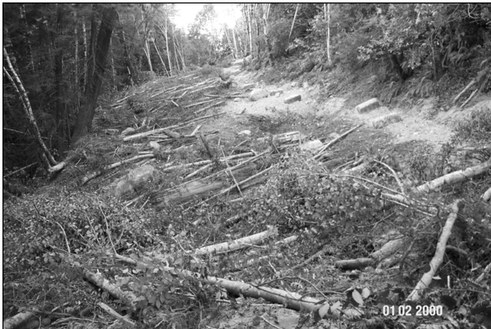
Figure X-D-27. Site # 2, 1312 Lower Road, after excavation. This picture was taken from the same viewpoint as above. The unstable road fill has been completely excavated. Straw mulch and seed had not yet been spread in this picture (note straw bales near former cutbank).
