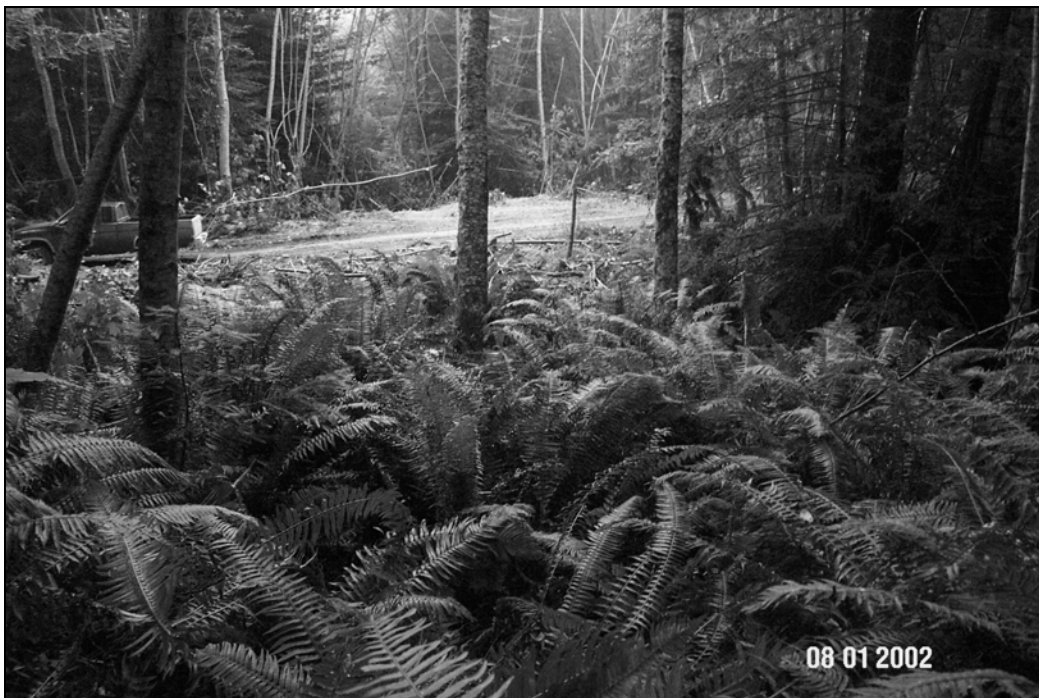
Figure X-D-9. Site # 12, 1300 Road, before excavation. This picture was taken 20 feet above the top of the stream crossing and along the left bank, looking downstream. The stream crossing has been brushed out and is ready to be excavated.
