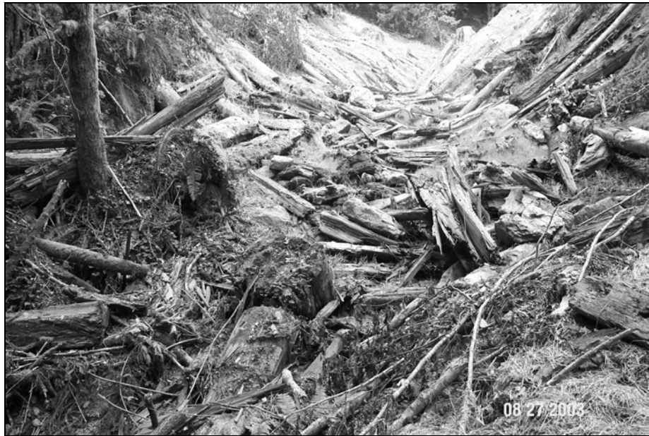
Figure X-D-21. Site # 3, 1311 Road, after excavation. This picture was taken near the same location as the previous photo. The stream crossing has been excavated and an abundance of woody debris has been redistributed along the banks and the channel.
