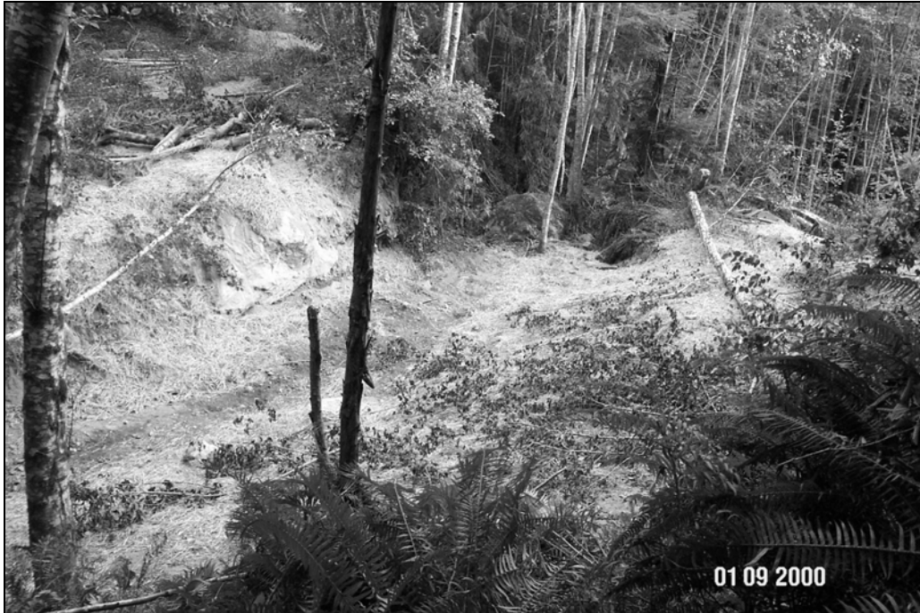
Figure X-D-8. Site # 8, 1300 Road, after excavation. This picture (and Figure X-D-7) was taken 30 feet up the right bank, near the right hinge line of this stream crossing. The stream crossing has been excavated, mulched and seeded. Note location of the two trees for reference.
