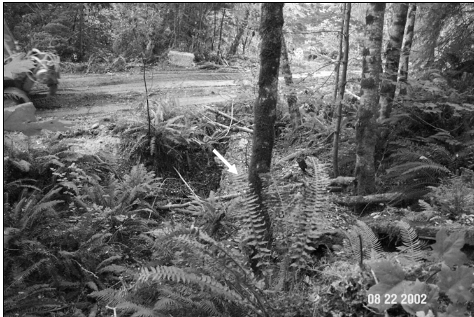
Figure X-D-13. Site #11, 1305 Road, before excavation. This picture was taken 30 feet above the top of the stream crossing and along the left bank, looking downstream. The stream crossing has been brushed out and is ready to be excavated. A large “Humboldt” log is visible just left of the mossy alder tree in the right-center portion of the picture (see arrow).
