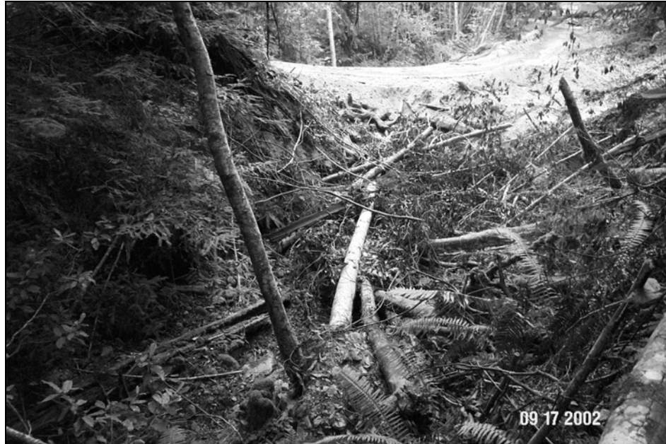
Figure X-D-4. Site #8, 1300 Road, before excavation.
