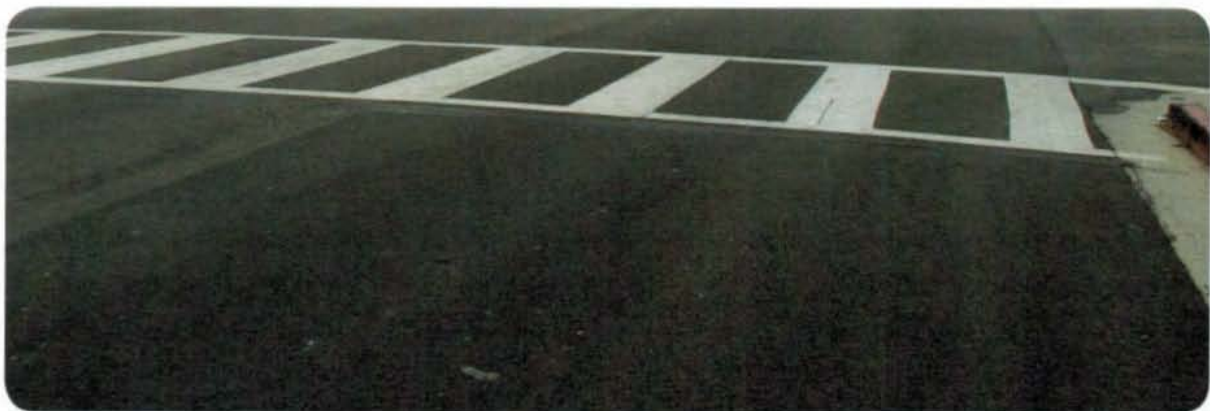
Figueroa - 42nd to 43rd, Pavement Condition 100, Grade A
