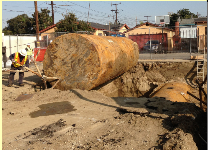
Photo 2: UST Removal in progress
