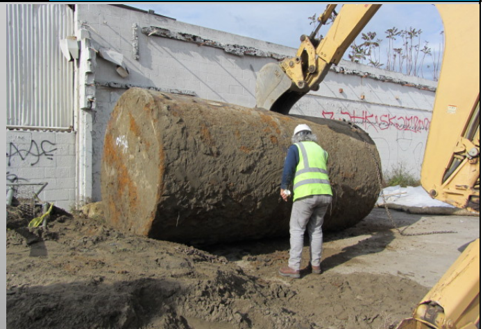
Photo 1: Removal of a gasoline UST
