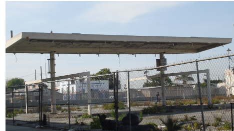
Photo 3: Abandoned UST Site
