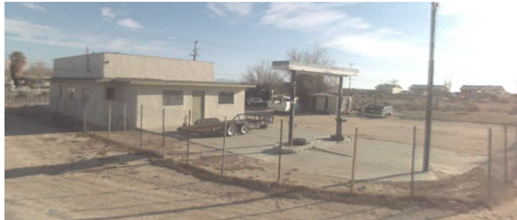
OPEN - SITE ASSESSMENT
