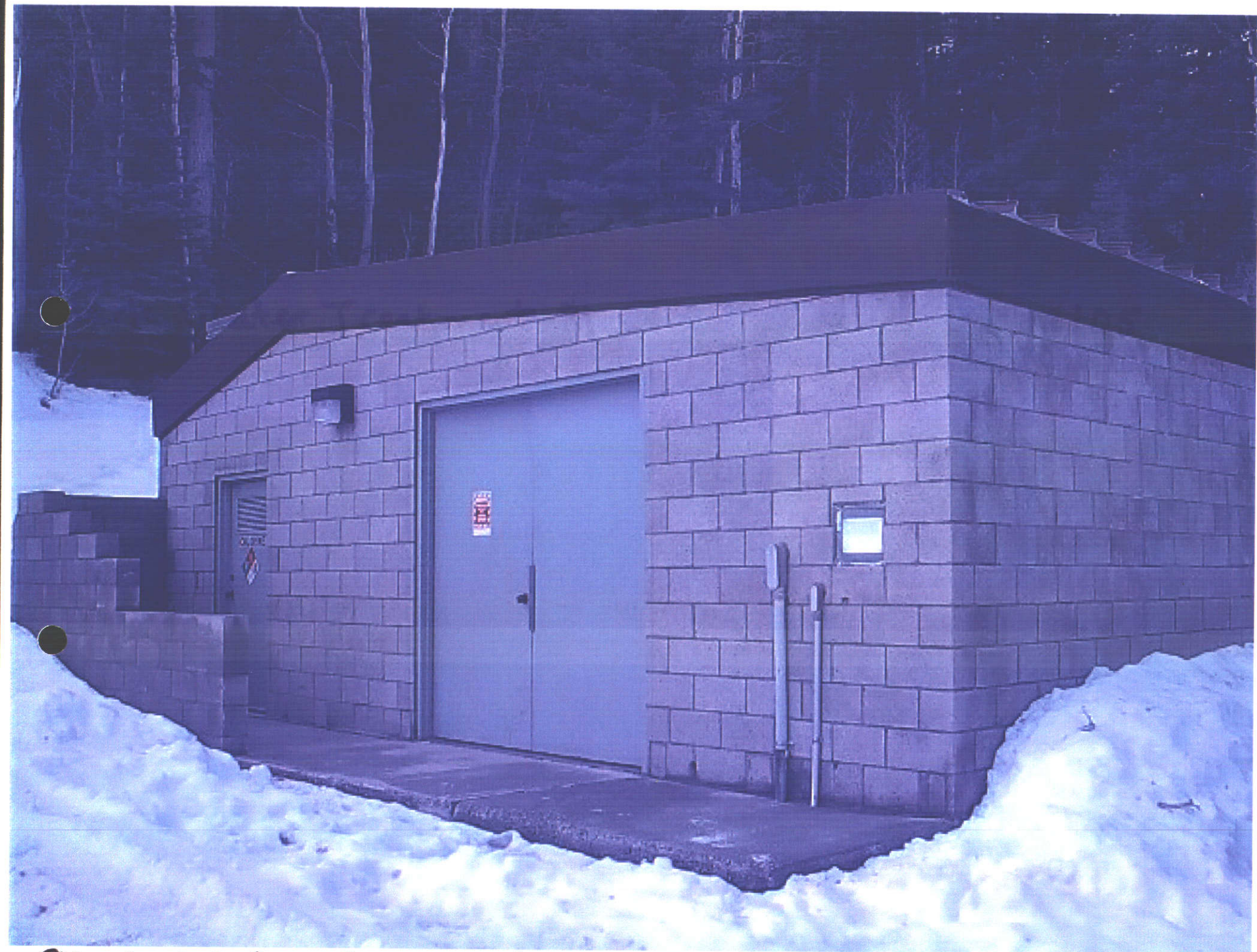
Clark Water Treatment Plant
