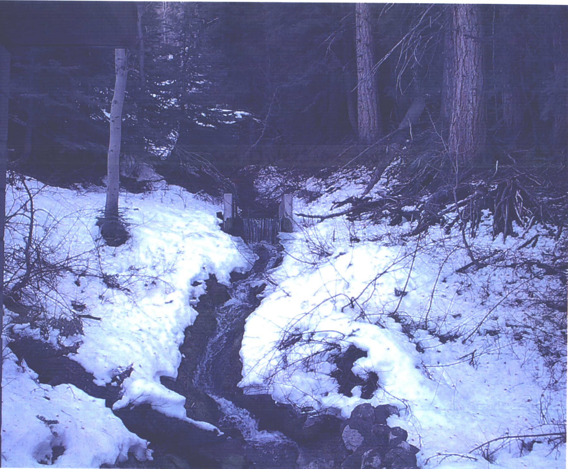
Unnamed Creek - Petersen Diversion looking upstream 12/05
