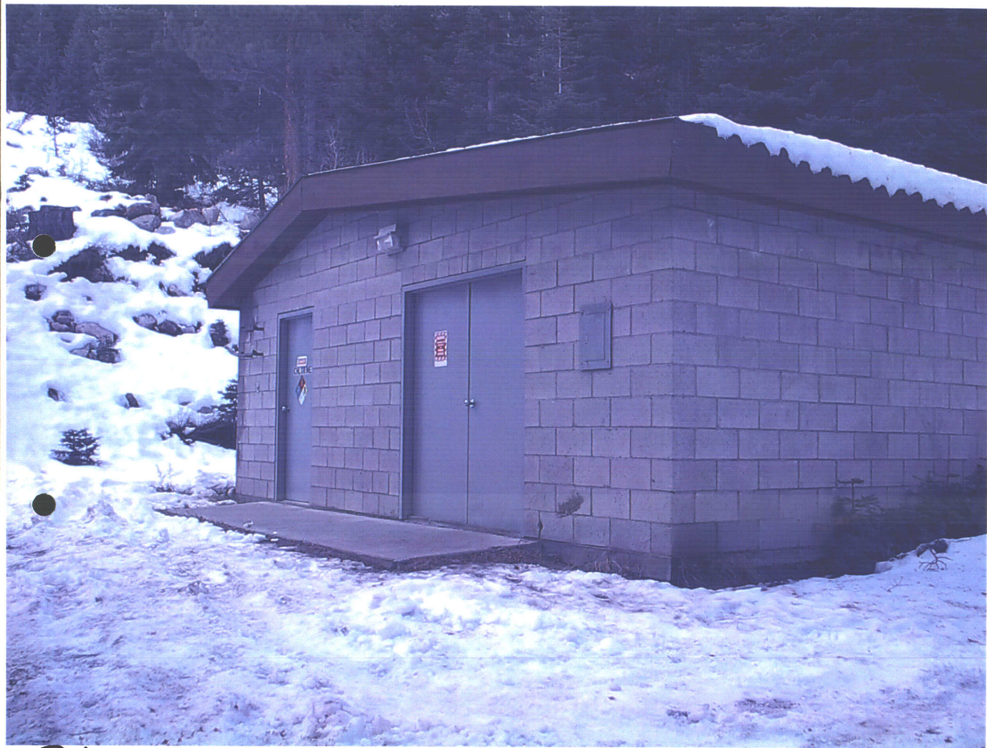
Petersen Water Treatment Plant
