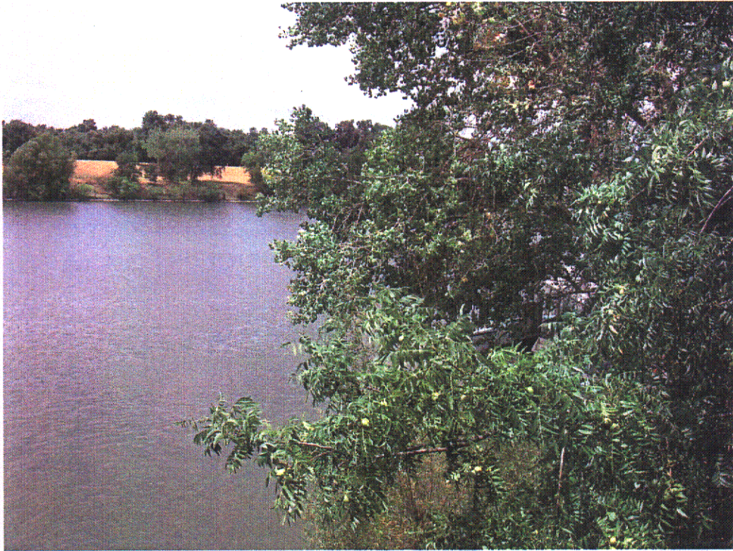
POINT 6 - Riverside Pumping Plant – View North
