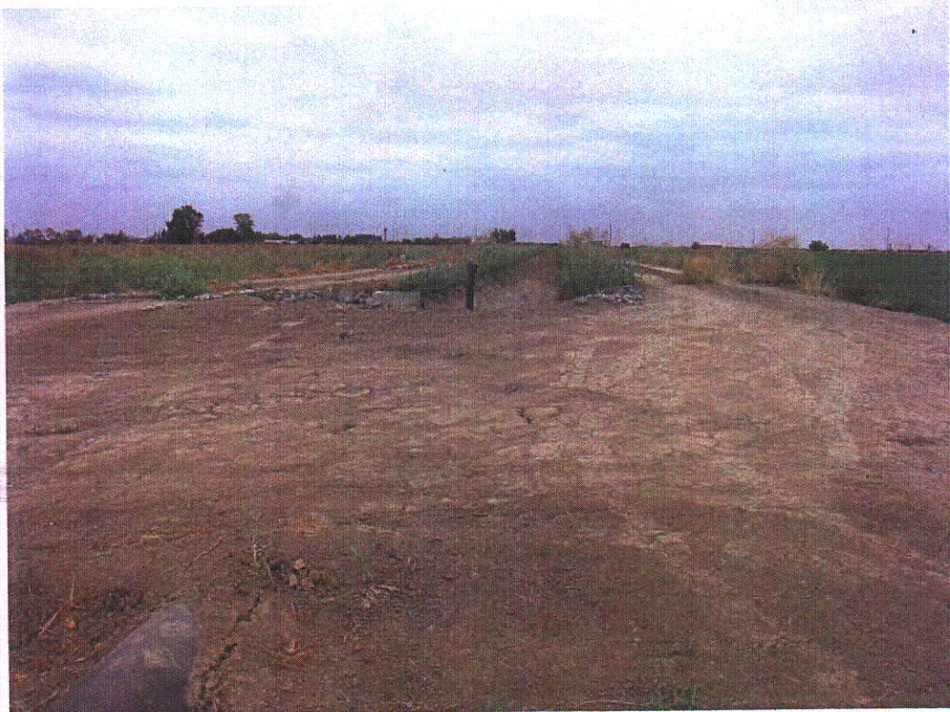
POINT F to POINT G - Airport/Bayou Lift Station – View North
