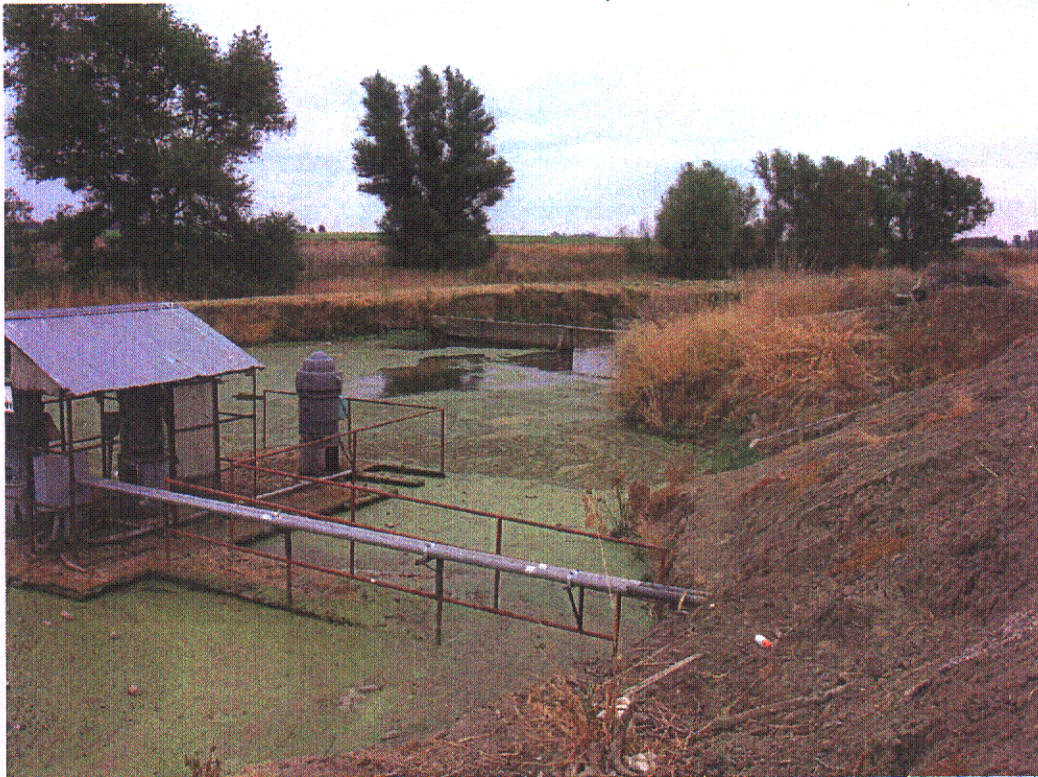
POINT E to POINT 2 - Pullman Lift Station – View Northeast
