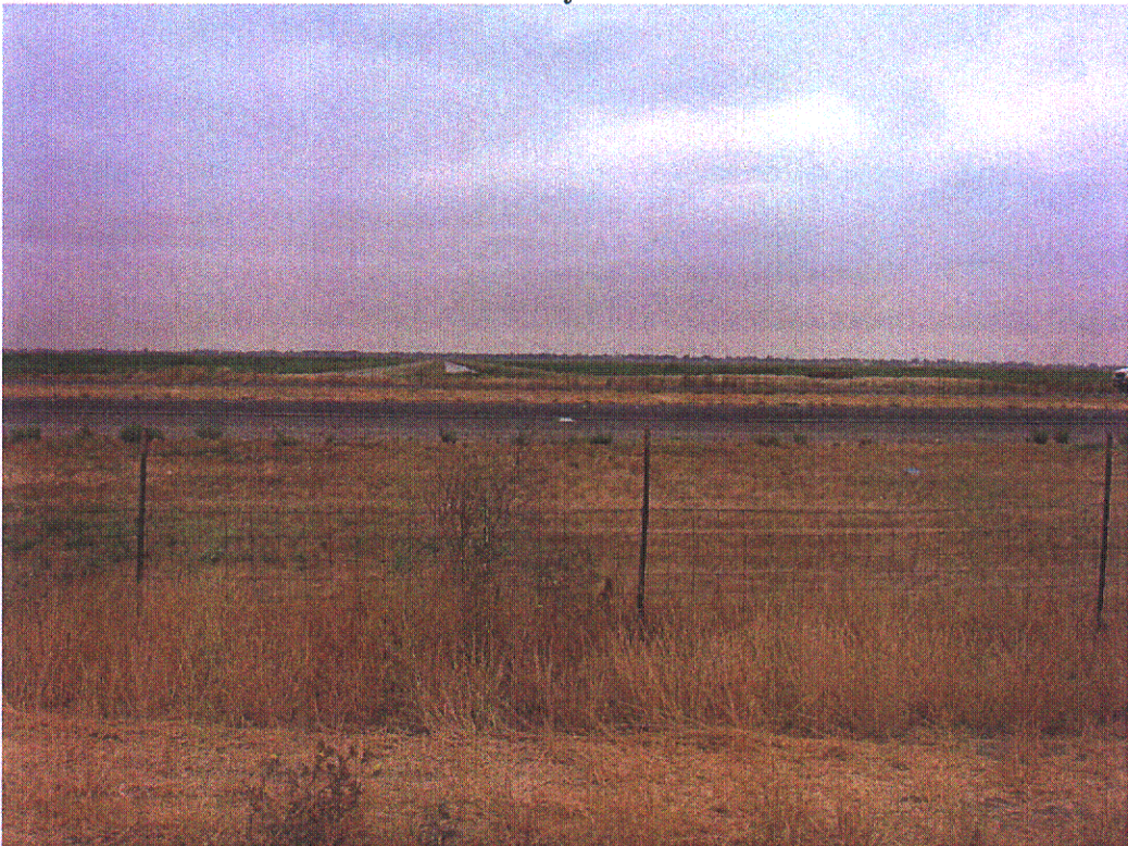
POINT E to POINT F - County Line Lift Station – View West
