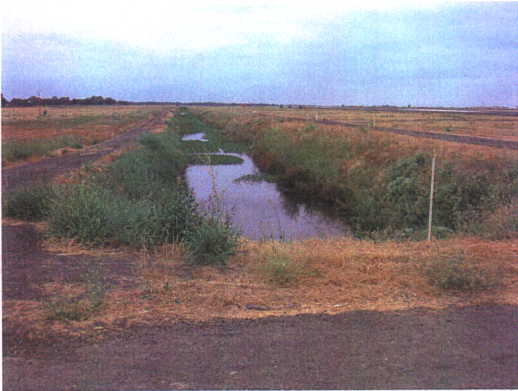
POINT F to POINT G - Airport North Drain Pump – View North
