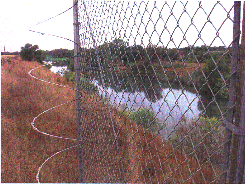
POINT A - Bennett Pumping Plant - Southwest
