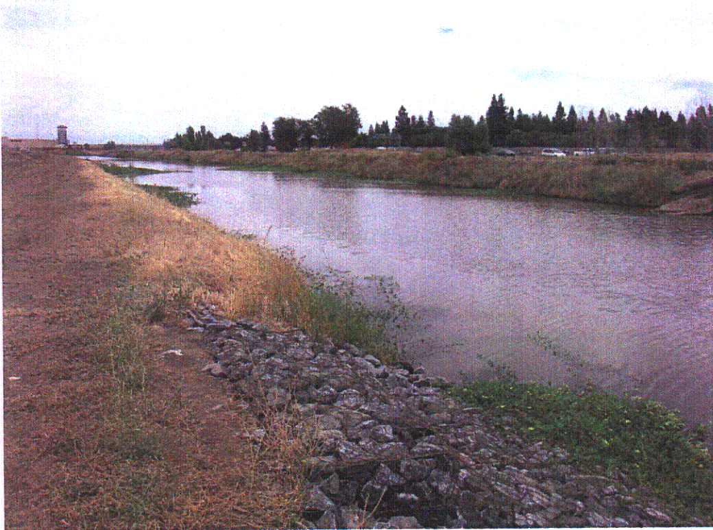
LNWI Intake (East Drainage Canal) – View East
