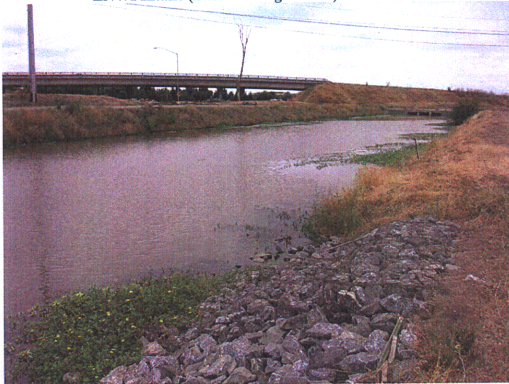
LNWI Intake– View West
