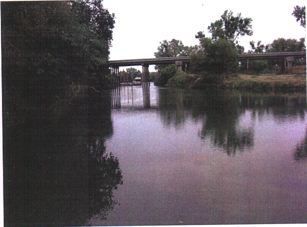
POINT 1 - Verona Pump Station – View Southwest
