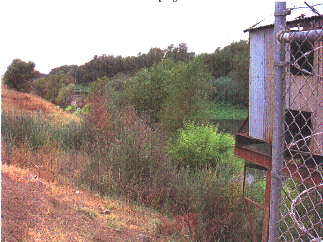
POINT B - Northern Pumping Plant – View Southwest
