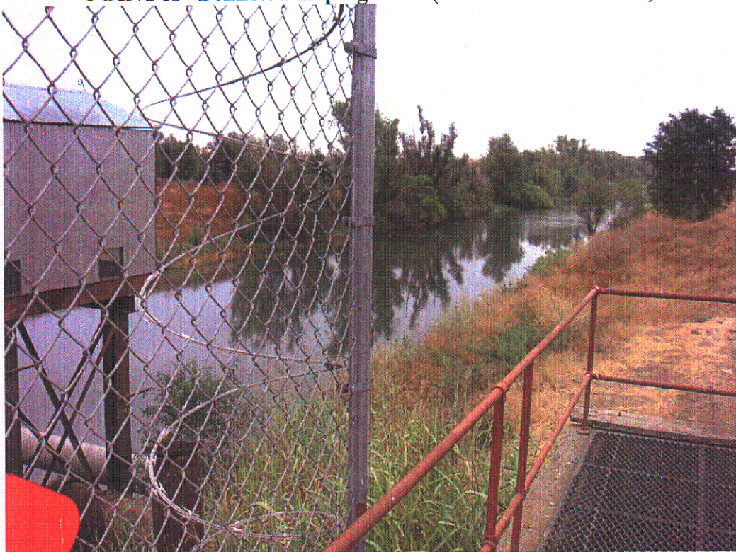
POINT A - Bennett Pumping Plant – View Northeast
