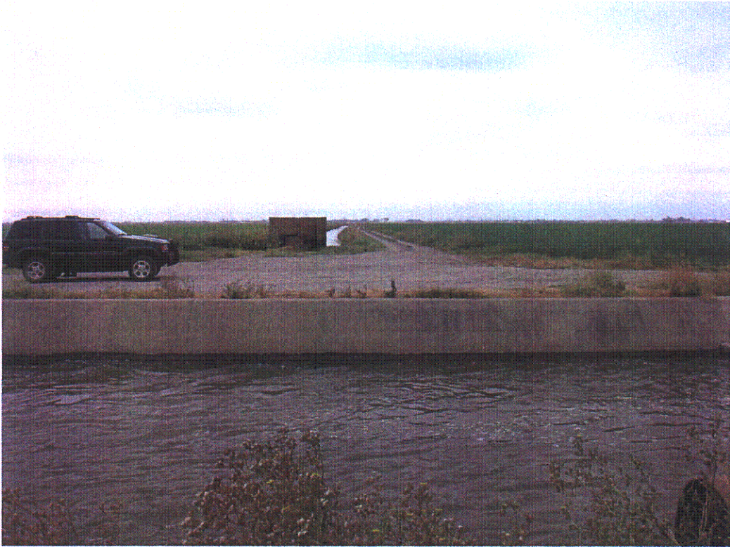
POINT E to POINT F - County Line Lift Station – View East
