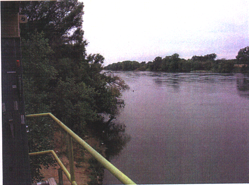
POINT 3 - Elkhorn Pumping Plant – View South
