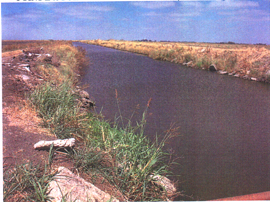
POINT E to POINT F - Elkhorn Lift Station – View North
