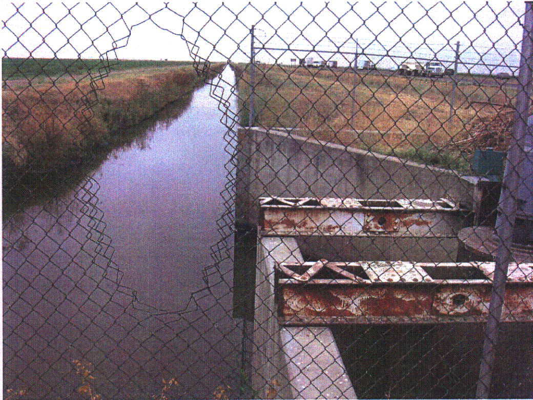
POINT E to POINT F - County Line Lift Station – View South
