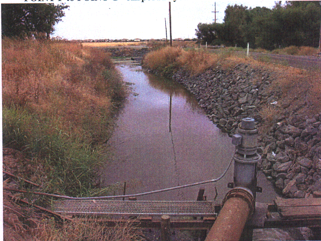
POINT F to POINT G - Rosa Drain Pump (West Drainage Canal) – View East
