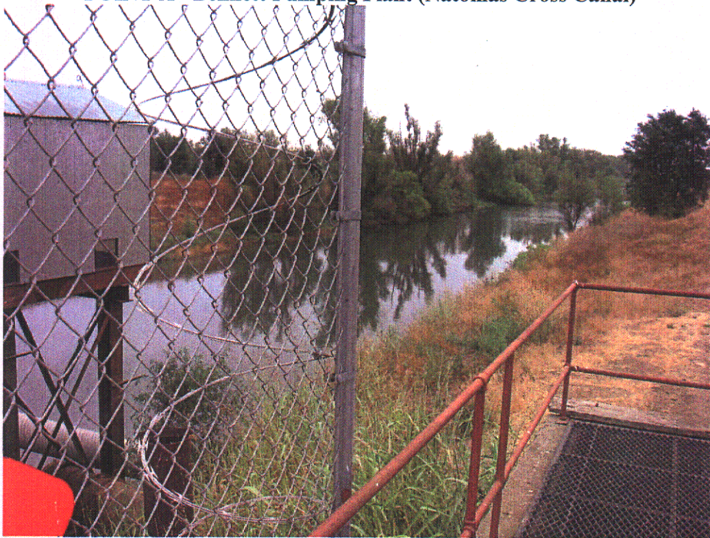
POINT A - Bennett Pumping Plant – View Northeast
