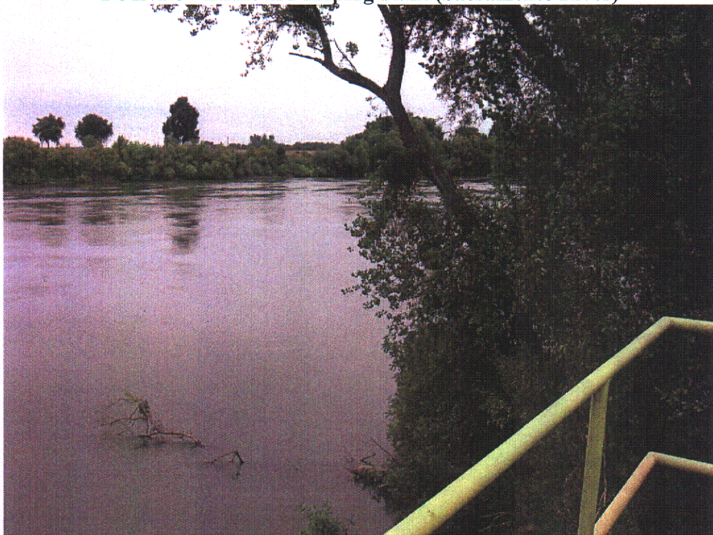
POINT 3 - Elkhorn Pumping Plant – View North
