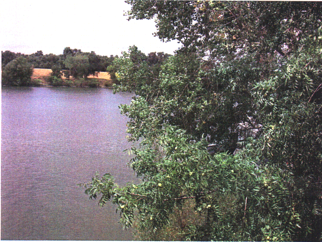
POINT 6 - Riverside Pumping Plant – View North
