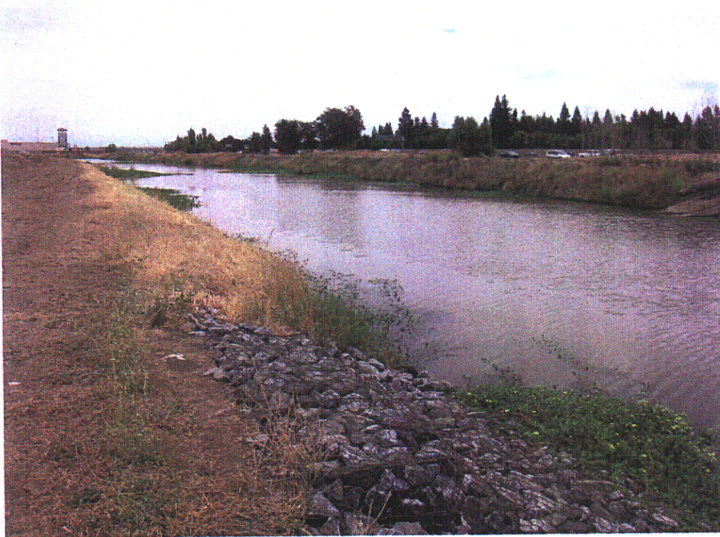
LNWI Intake (East Drainage Canal) – View East
