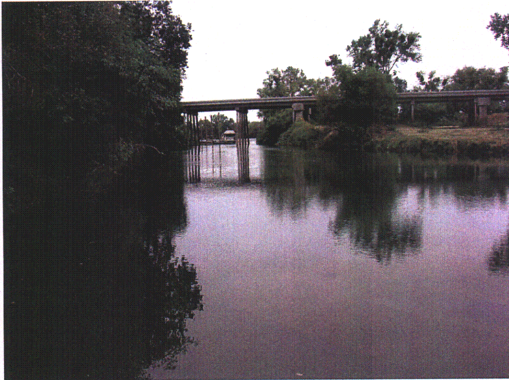
POINT 1 - Verona Pump Station – View Southwest
