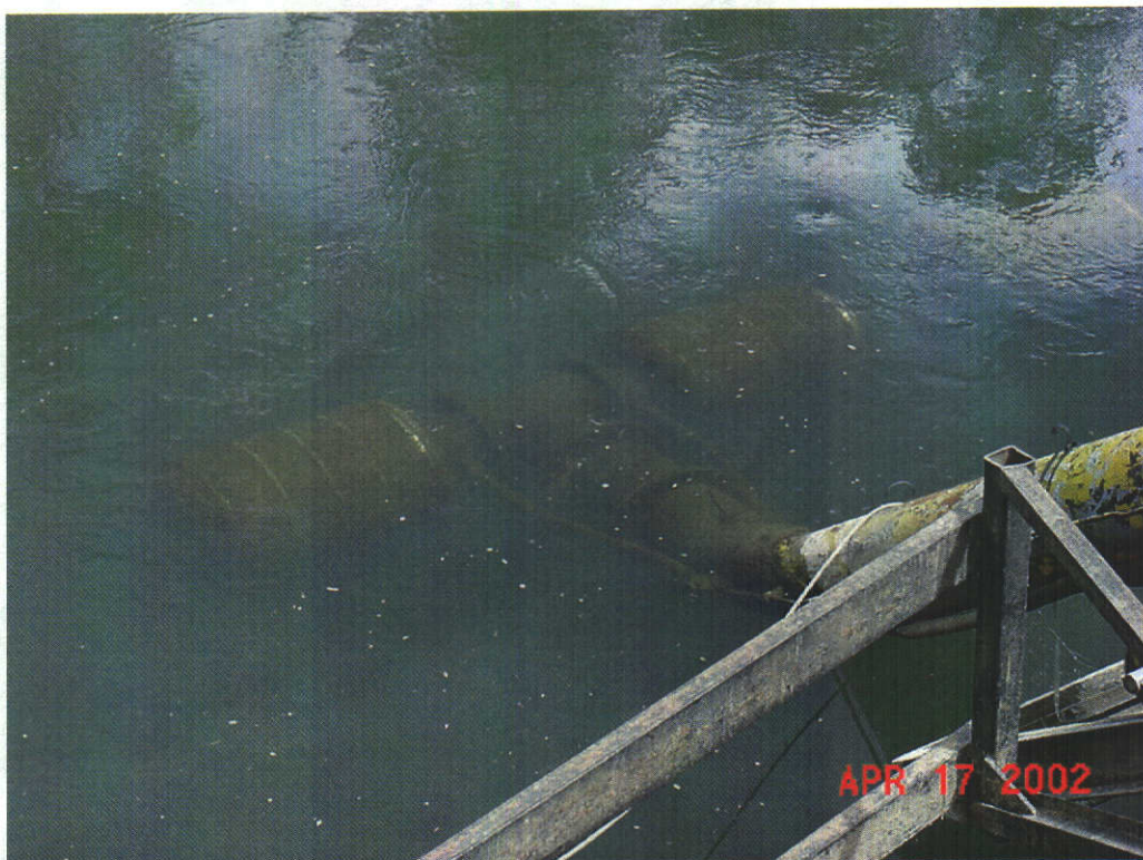
Fish screens on surface diversion
