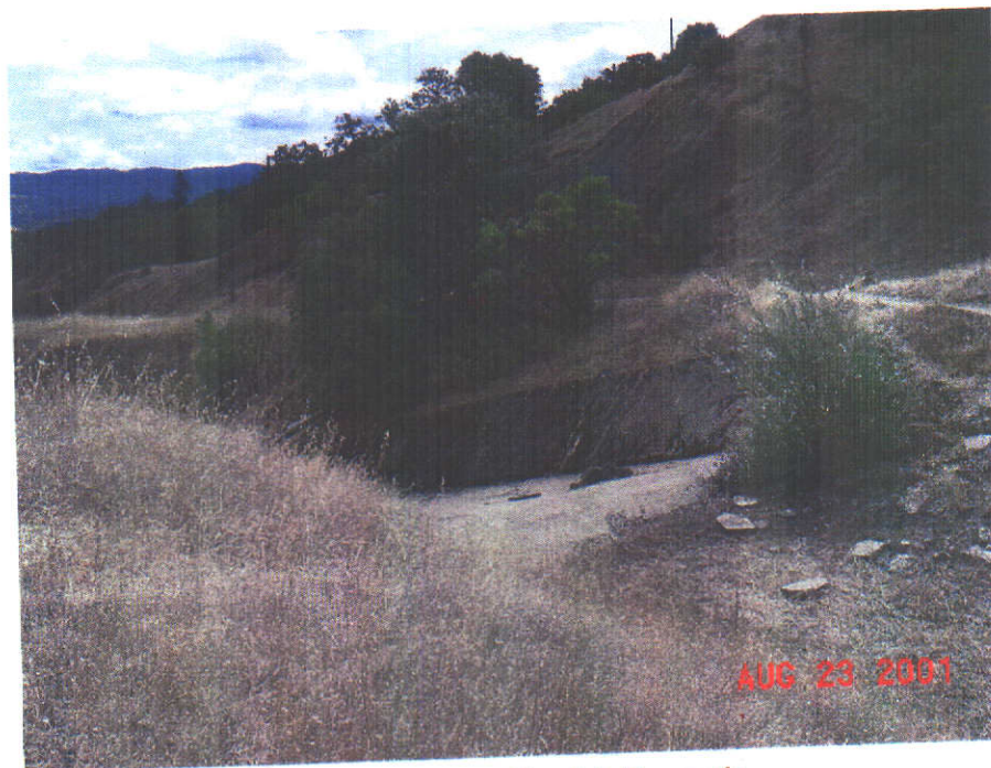
Spillway at Round Mountain Reservoir.
