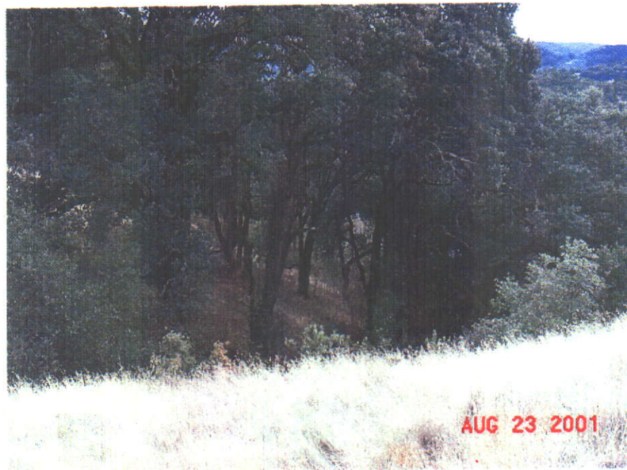
Deep ravine immediately above the sump. The ravine has steep sides and creates a channel for the runoff.
