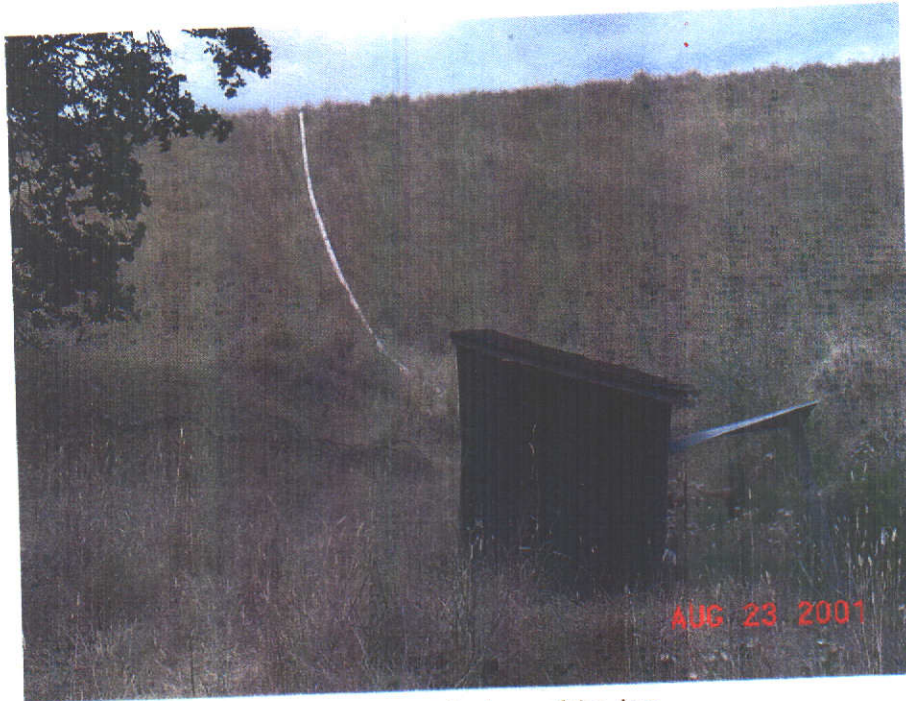
Pump house at the base of the dam.
