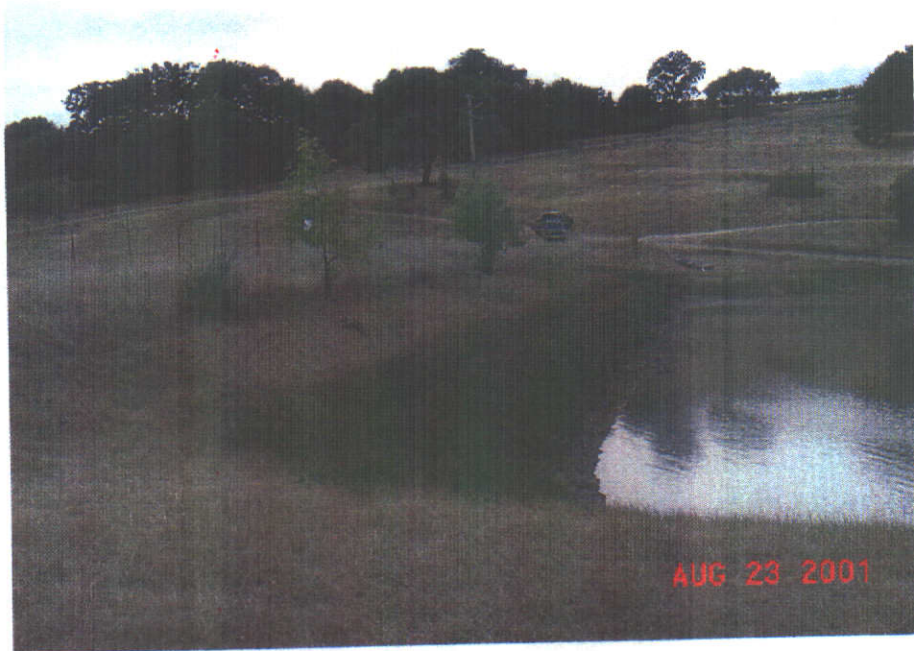
The dam at the Lower Reservoir looking to the west.
