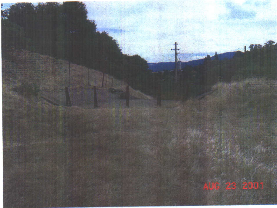
The spillway at the Lower Dam.
