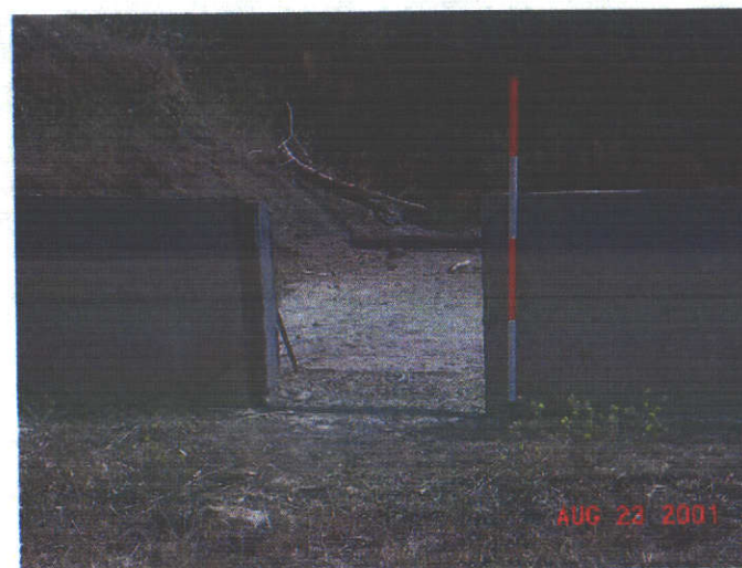
Spillway in the dam at the "Back" Reservoir.
