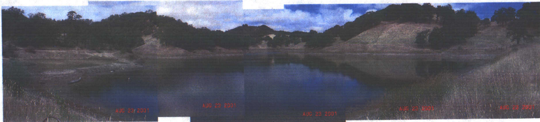
Round Mountain Reservoir viewed from the dam.
