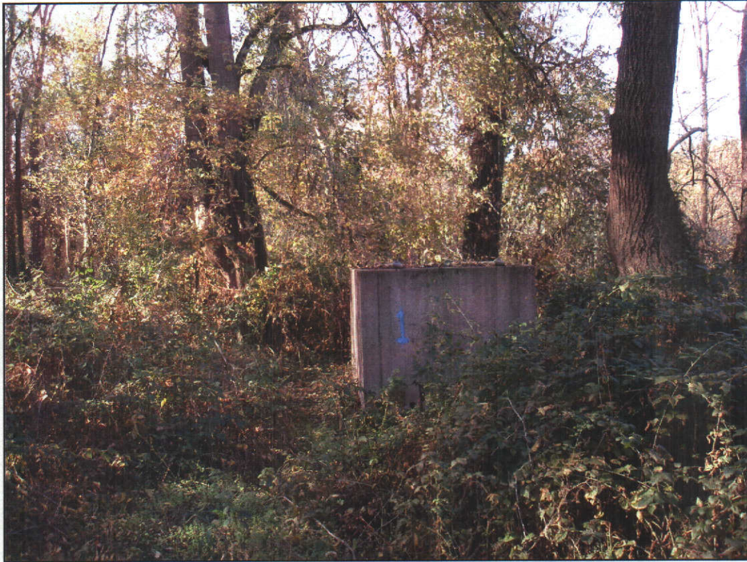
Photo of the existing District Well 1.
