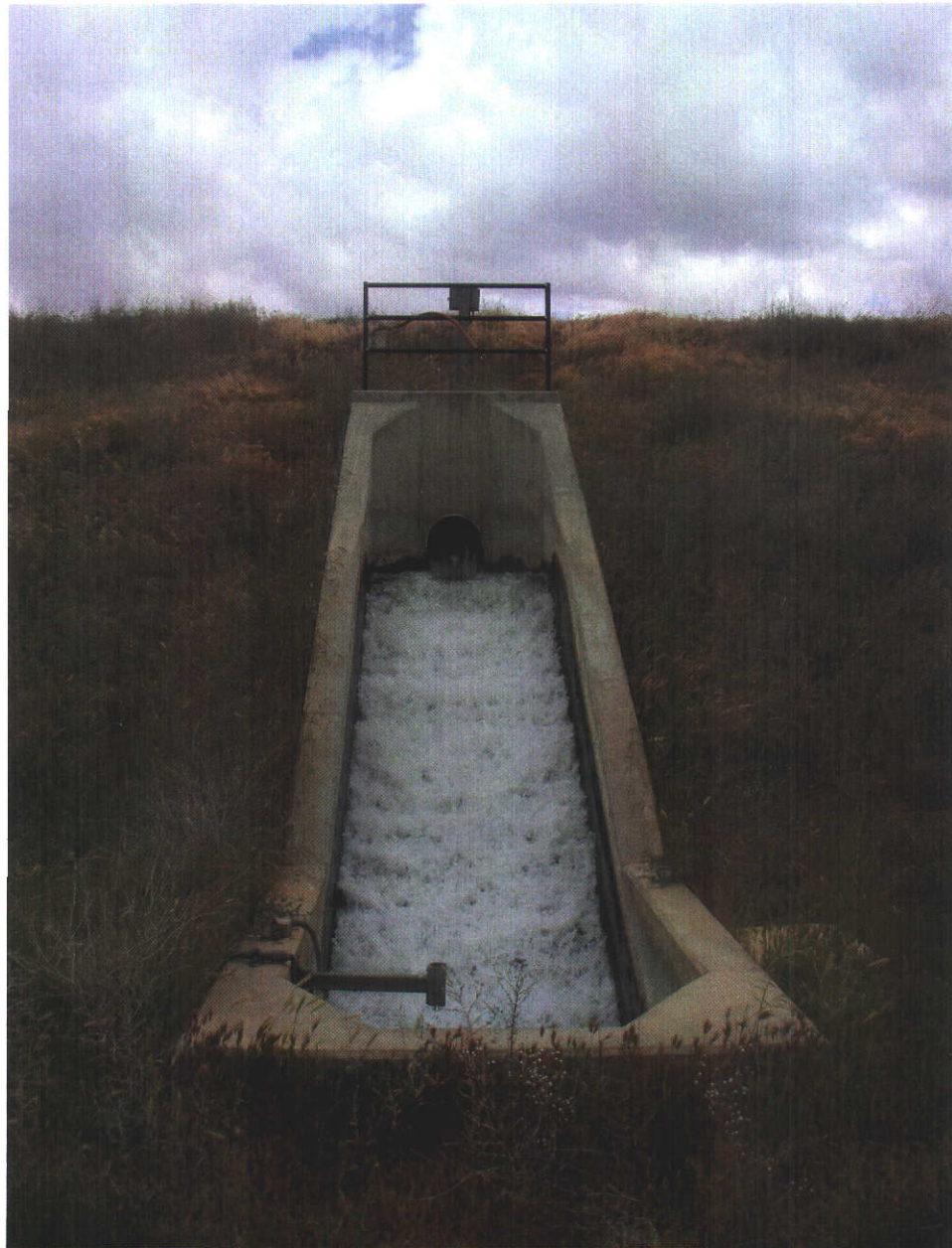
DP001 - Upstream of the Discharge Point (Outfall, Looking North)
