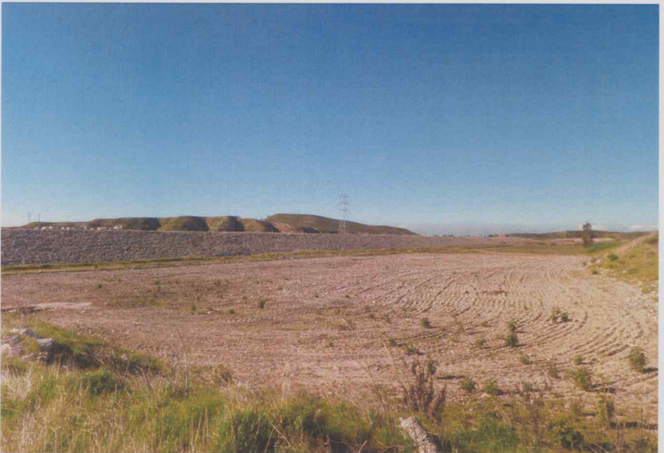
Devil Canyon Recharge Facility, looking South-West.
