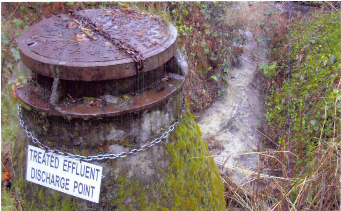
Photo 2: SMD 3 POD; February 10, 2012
