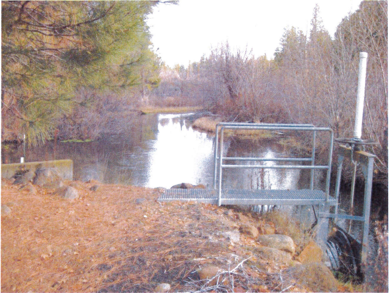
View of Fall Creek looking upstream from diversion dam (left dam abutment visible at left). Bypass control gate is at right (photo date December 2013).
