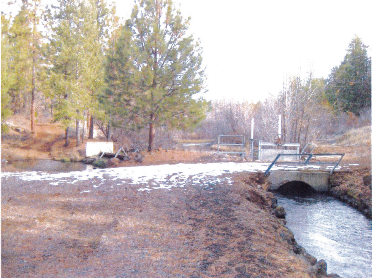
View of Fall Creek at point of diversion looking upstream. Diversion dam at left, conveyance canal and control gate at right. Photo also shows another control gate, located immediately left of the canal control gate, that is used to bypass Creek flows around the diversion dam (photo date December 2013).
