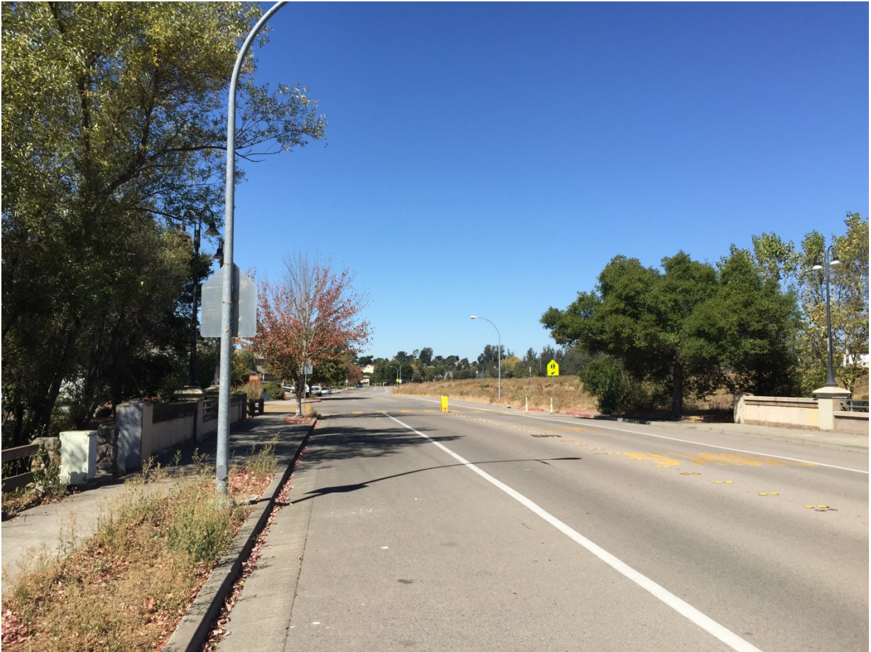
Figure 3- Corona Creek crossing
