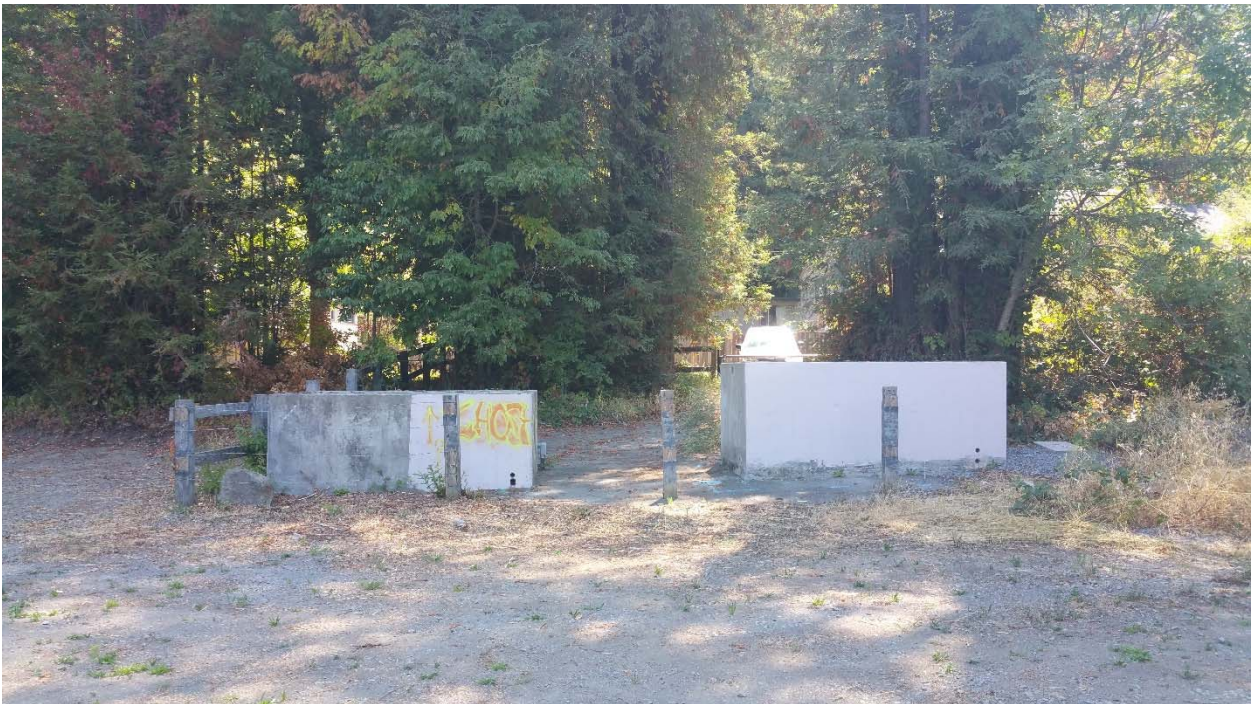
OCSD Well 2 on left, CMRPD Well 1 on right looking southerly away from Russian River.
