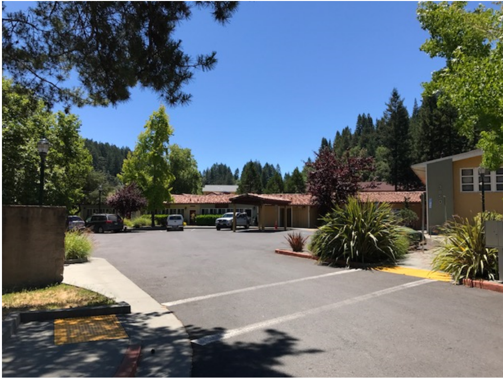
Harmony Village residential/commercial complex, entrance driveway
