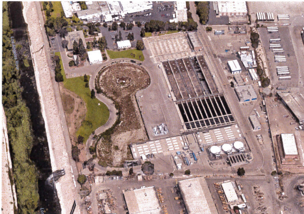
Figure 5: Ariel of LAGWARP and Discharge Point
